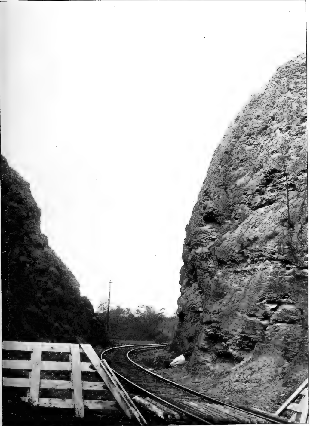
Rock cut in Cashaqua shales. Cashaqua creek
