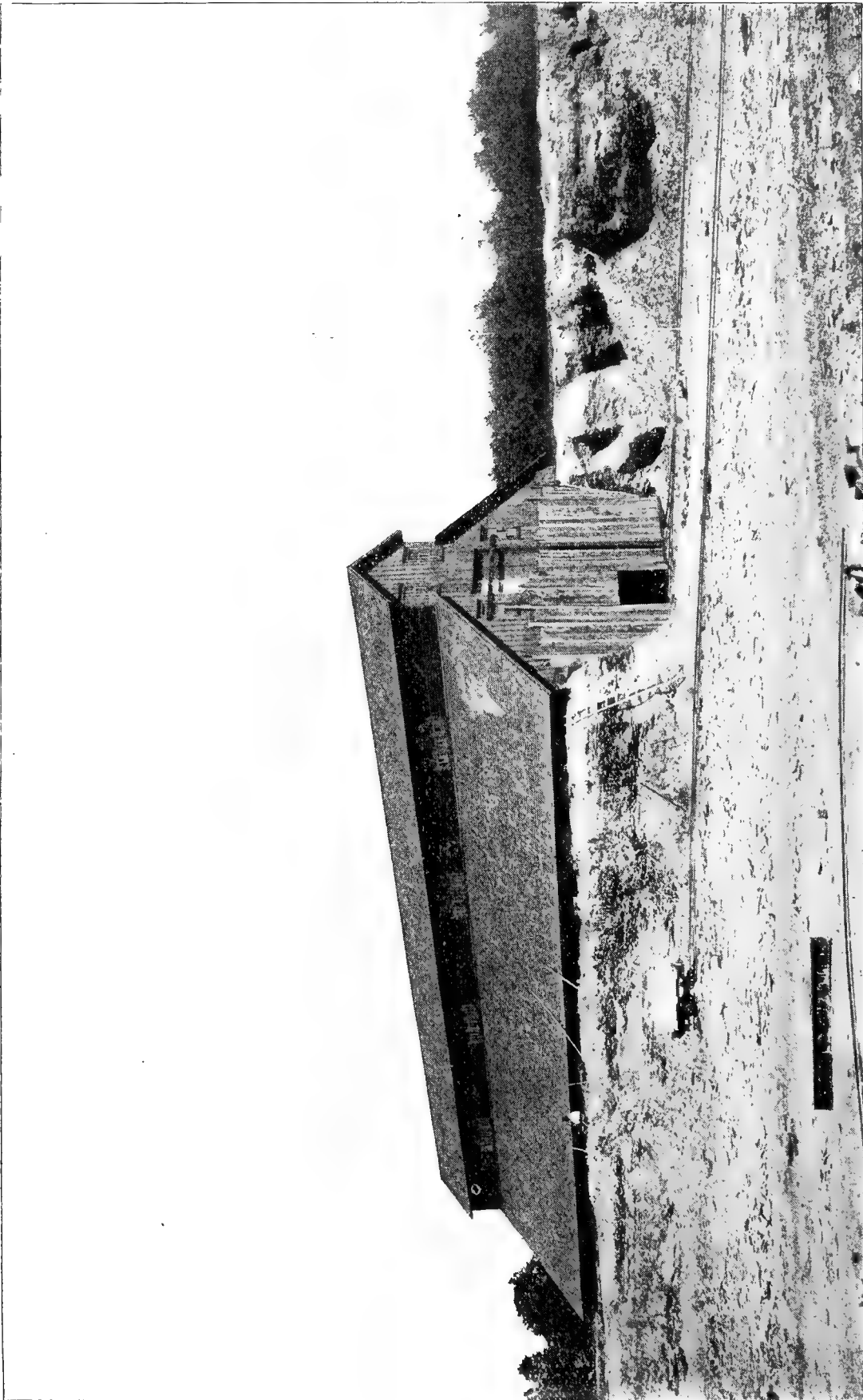
H. Ries photo. Shale bank, J. Lyth & Sons, Angola. The roofed over portion is worked in winter.
