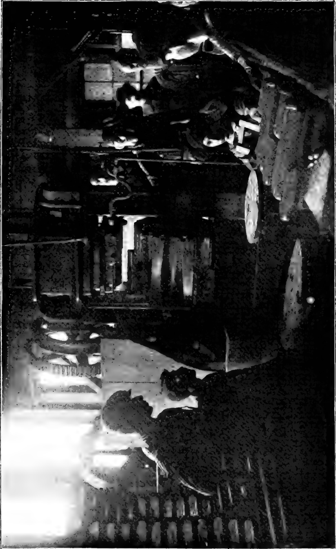
H. Ries photo. Rear view of roofing tile press, showing the green tile (a) which have just been received from it.
