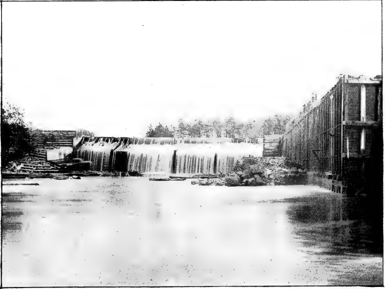
A. Dam on Schroon river at Warrensburg, with flash boards in place.
