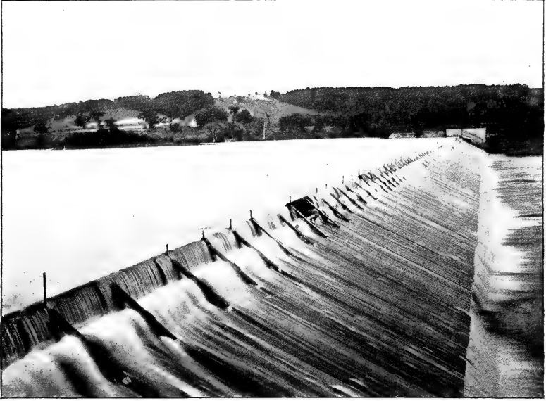
A. The dam at Mechanicville with flash boards in place.
