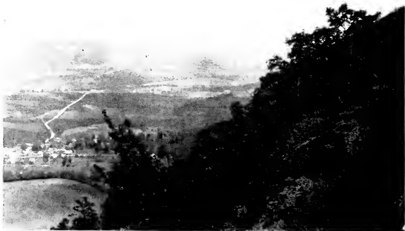
Figure 52. The village of Copake Falls as seen from Washburn Mountain; the village is about 200 meters below the point from which the picture was taken. Note the lichens growing on the otherwise bare rocks in the right foreground.
