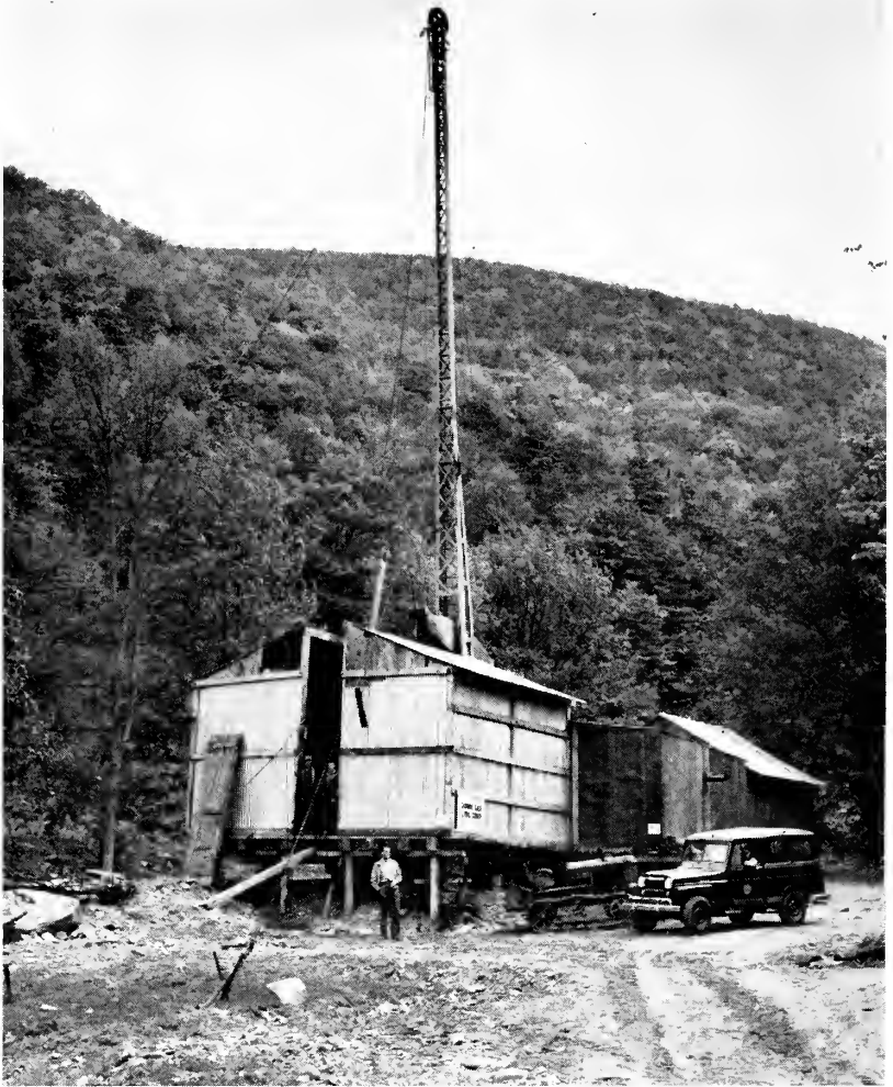
Members of the Geological Survey, State Museum and Science Service, visit a rig which is drilling for gas or oil in the Catskill Mountains. Examination of the well cuttings assists in identification of the rock formations being penetrated. This aids the oil and gas industry in planning the location of future drilling sites.
