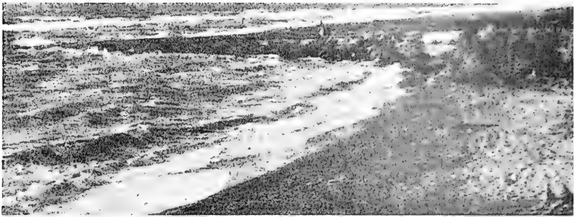
FIGURE 16. COAST EROSION LEEWARD OF GROIN AT BOVBJERG.
