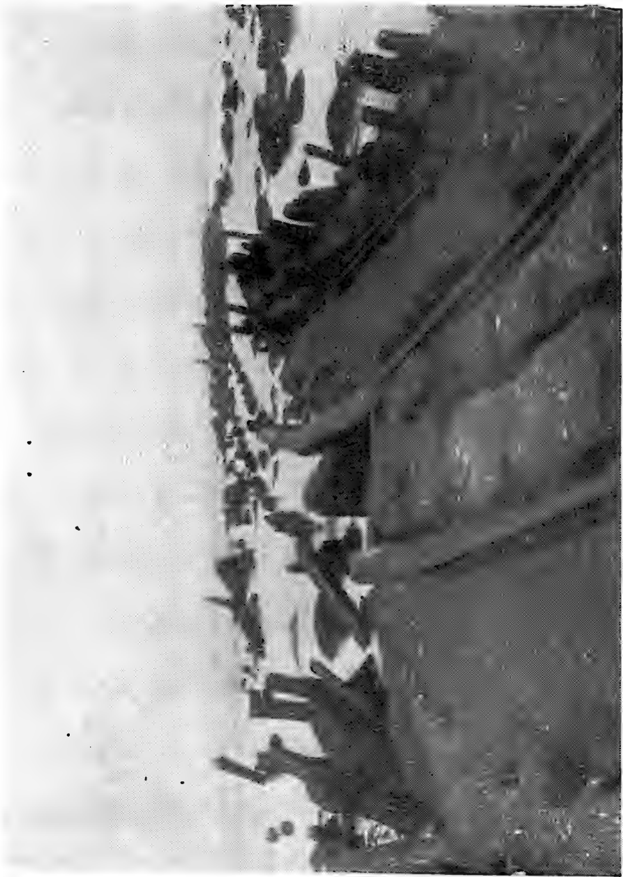
Figure 25. The north section of the connecting dam at Hook of Holland which was damaged and partially destroyed by high tides. Picture taken in August 1947 at half tide.
