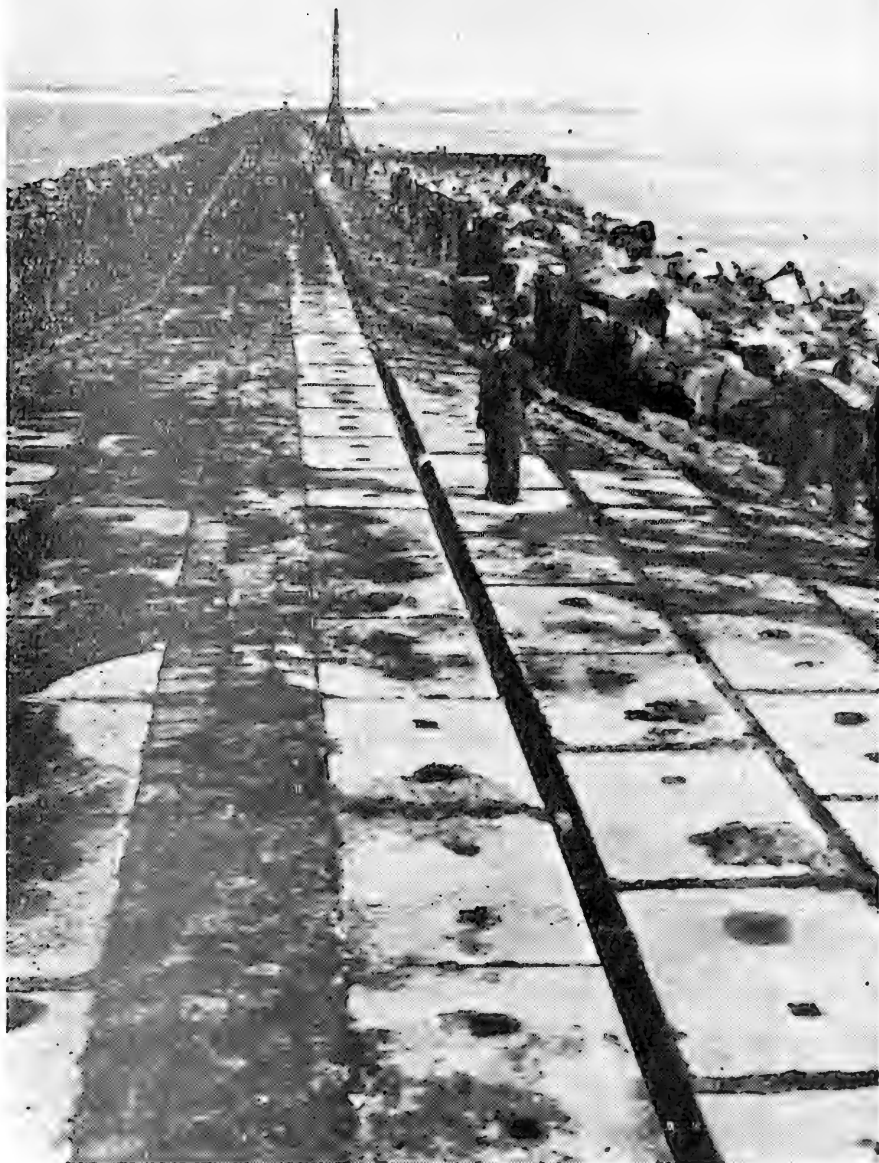
Figure 22. North pier, Hook of Holland. The conversion of the railroad track into track for trucks, consisting of concrete blocks and set stone with asphalt grouting carried out in 1948. The gutter to carry the lighthouse cable is in the center. In the foreground is the wide section near the foot of the lighthouse.
