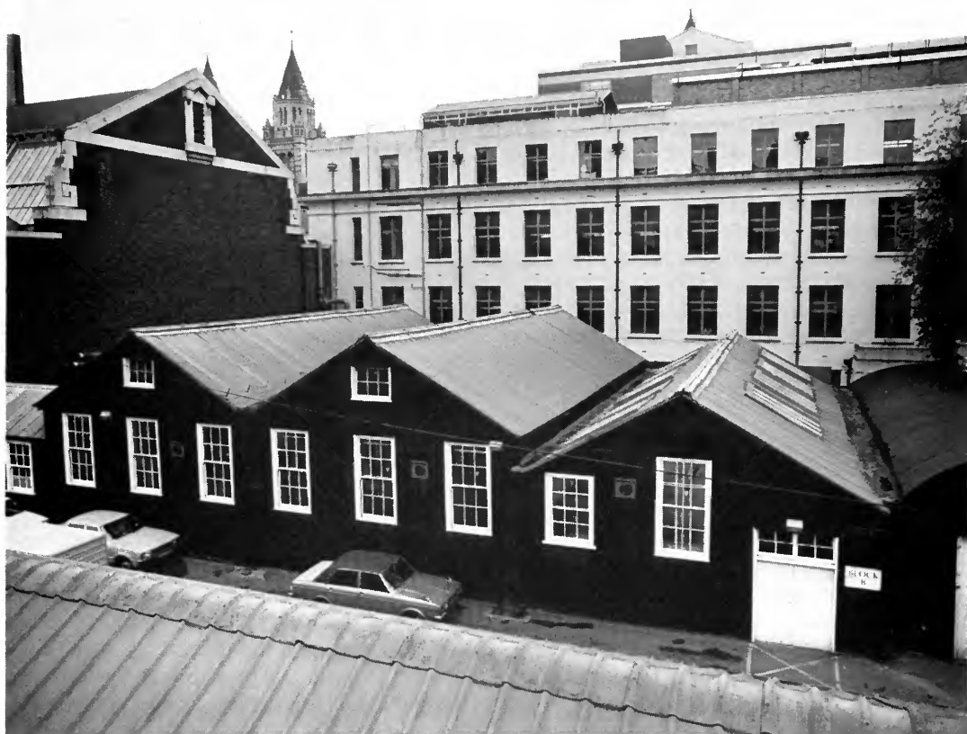
Plate 9 The Discovery Hut or Block B, showing the three main units of the building. In the left background is the west-central tower of the main Waterhouse Museum building. In the centre middle ground is the Department of Zoology Spirit Building, built between 1920 and 1930, and in the left centre the west end of the art deco Whale Hall, constructed between 1930 and 1934. The Entomology Block, begun in 1934 but, because of the war, not completed until 1952, is visible behind the Spirit Building.
