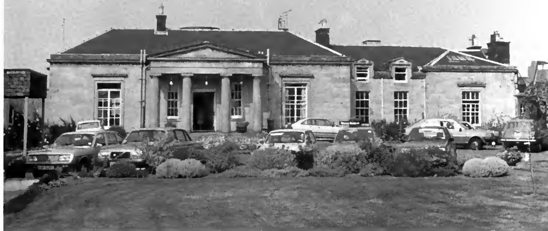
Plate 4 Challenger Lodge. Formerly Wardie Lodge, now St Columba's Hospice, northern Edinburgh.
