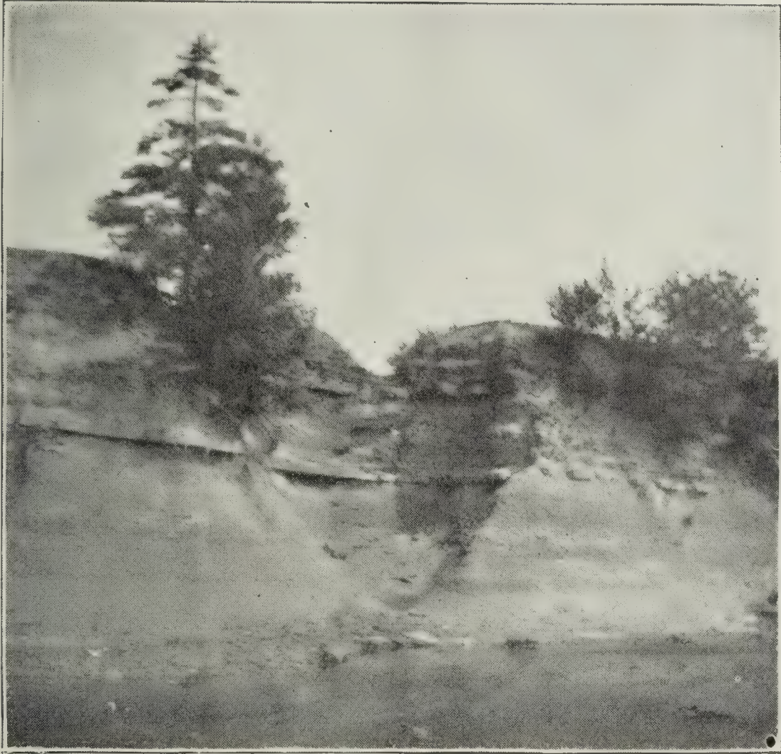
PLATE X.—View of the “corry” in Section 7, showing an example of gorge cutting in an early stage. The backward cutting of the falls produces the gorge, and the downward cutting of the stream the V-shaped trench seen above. The Encrinal limestone is seen near the middle of the cliff.
