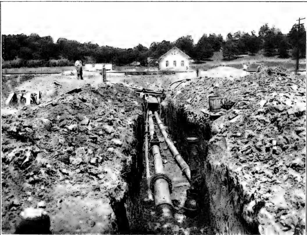
FIG. 7.—Three principal cast-iron pipe lines entering culvert beneath railway tracks. From left to right, the 4-inch clear-water supply, the 14-inch (reducing to 10-inch) reservoir supply, and the return 8-inch pond supply. In the foreground a valve box is seen; the valve controls an emergency "crossover" connection between reservoir supply and pond supply. (See text, p. 392.)
