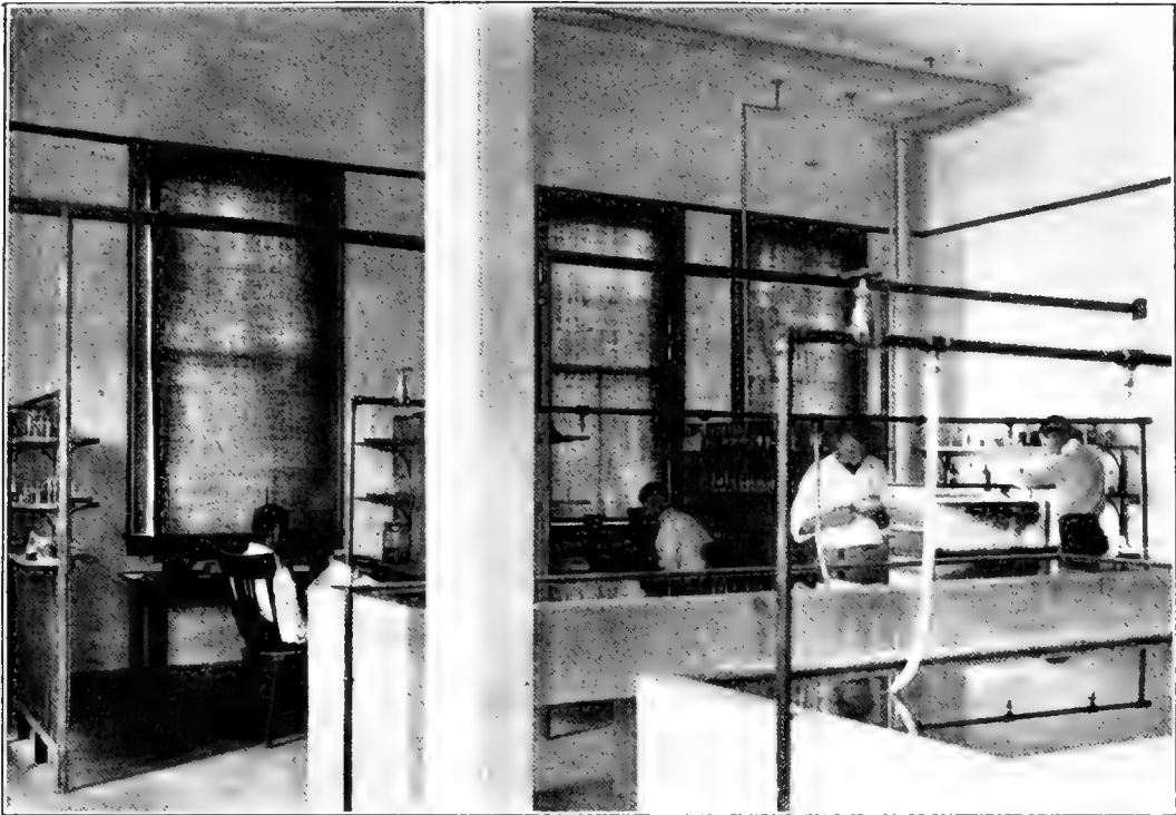
FIG. 6.—Interior of general laboratory, showing alcove arrangement and concrete tank tables.
