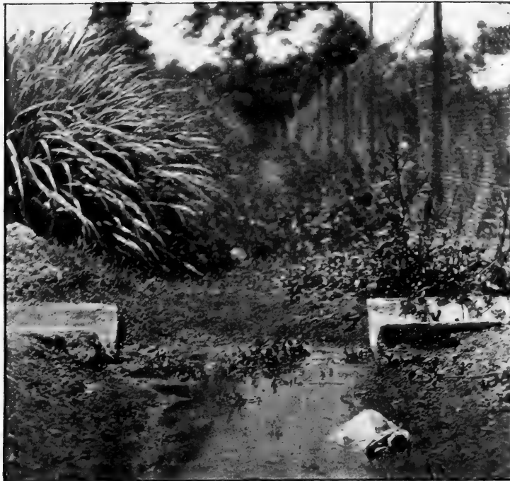
Fig. 1. Temporary pool at the open ends of a drain.
