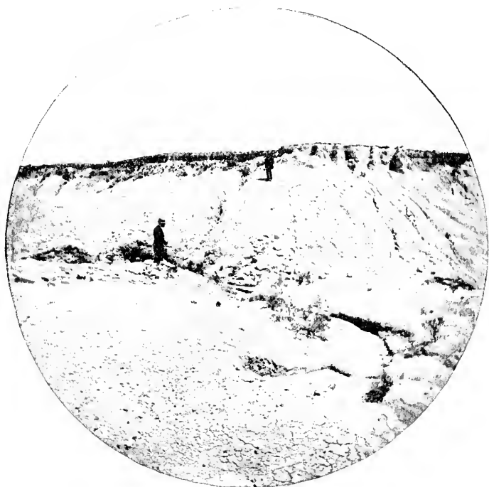
FIGURE 19.—Eastern End of Dike number 1. Showing that the dike did not reach the top of the bluff.
