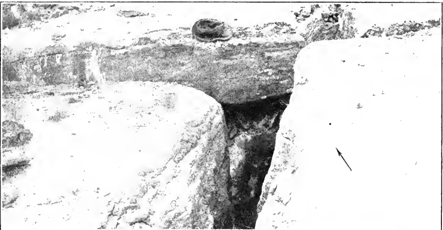
FIGURE 2.—AN ENLARGED JOINT CAVERN
