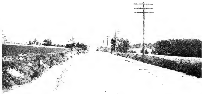
FIG. 8.—Type of improved sand-clay roads that are being built in the county.
