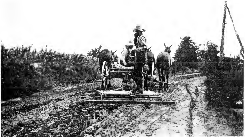
FIG. 5.—This scraper is being used quite commonly to put the roads in better shape
