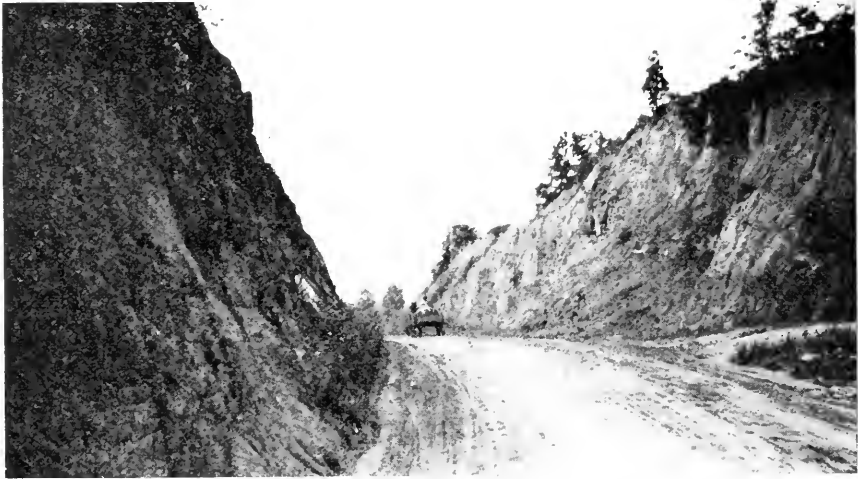
FIG. 4.—A modern type of sand-clay road that is being constructed in parts of the county
