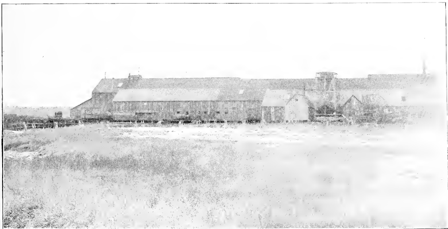
REAR VIEW OF CANNERY AT KUSSILOF, COOK INLET.
