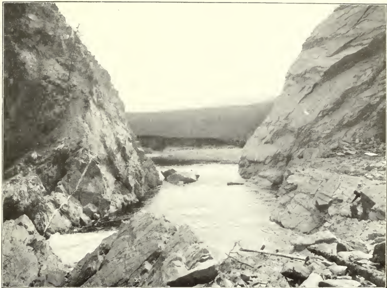
A. ARTIFICIAL CUT-OFF IN SCHIST ON NORTH FORK OF FORTY MILE.
