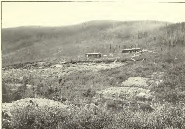
A. WASHING THE OVERBURDEN FROM THE GOLD-BEARING GRAVELS, WADE CREEK.
