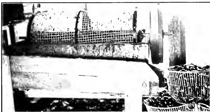
FIG. 226.—Revolving screen cylinder in tank of water used for final cleansing of mussels. Wire baskets for holding mussels are shown at right.
