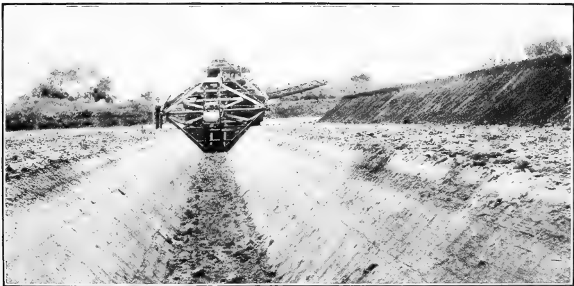
FIG. 2.—CONVERTIBLE TRENCH AND OPEN DITCH EXCAVATOR.
