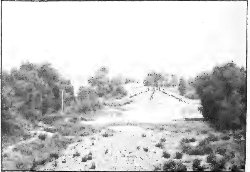
FIG. 2.—CONSTRUCTION OF LEVEE SHOWING SLOPE BOARDS. LEVEE CONSTRUCTION BY HYDRAULIC-FILL METHOD.
