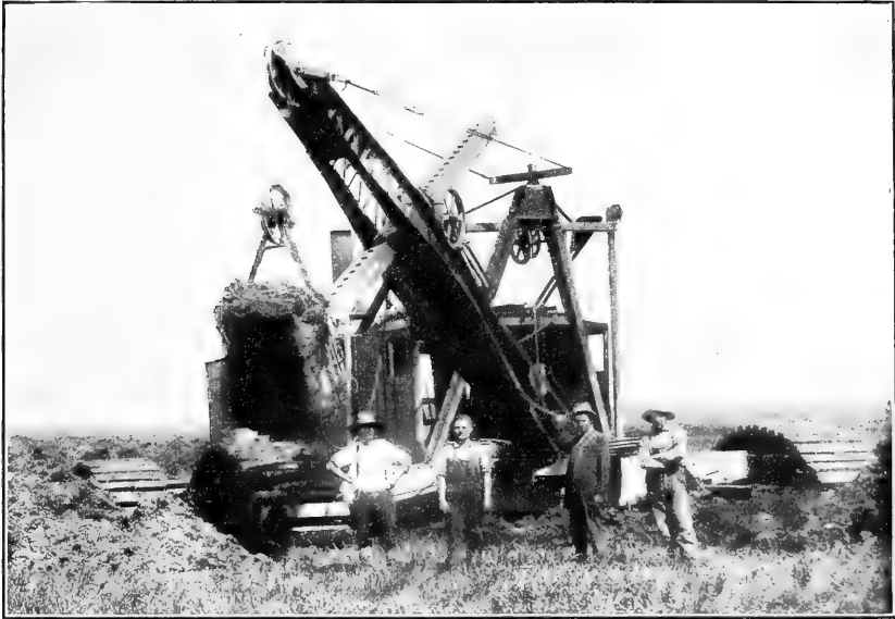
FIG. 1.—A 1-YARD DRY-LAND DIPPER EXCAVATOR MOUNTED UPON CATERPILLAR TRACTORS.
