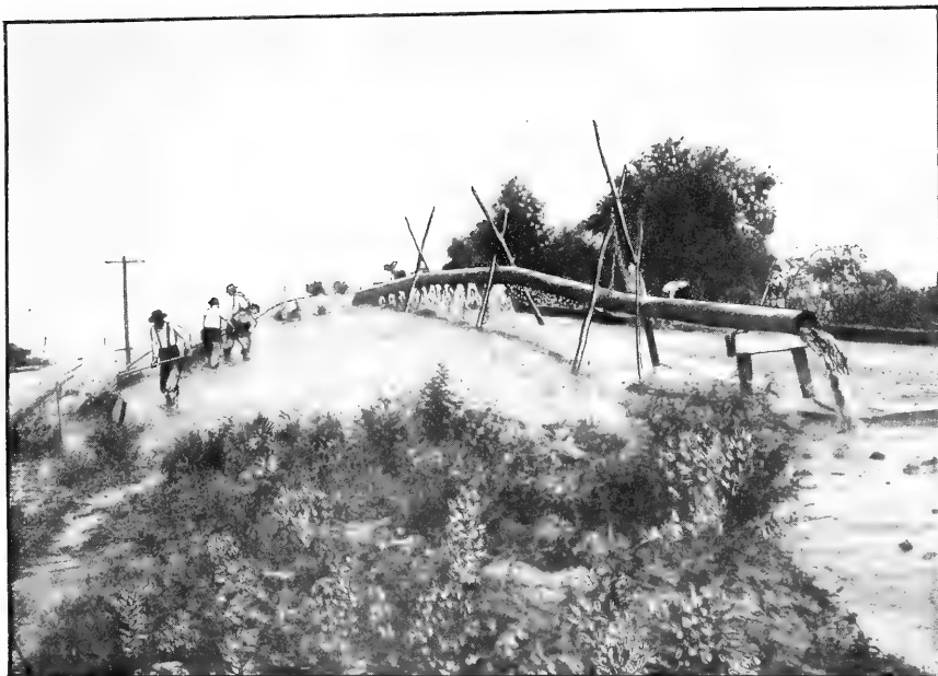
FIG. 1.—HYDRAULIC-FILL LEVEE CONSTRUCTION SHOWING METHOD OF FORMING LEVEE SLOPES.
