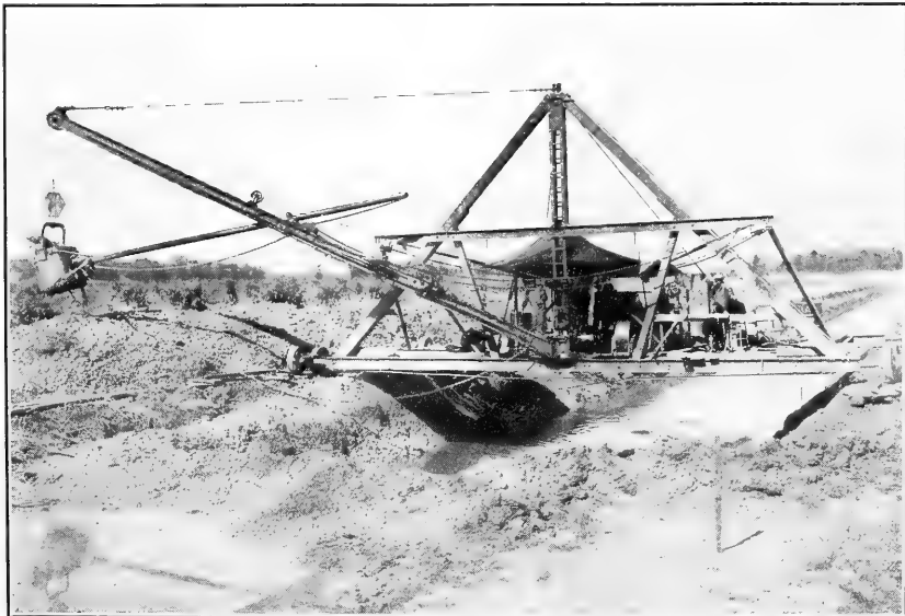
FIG. 2.—A 1-YARD DRY-LAND DIPPER EXCAVATOR MOUNTED UPON TRUCKS.
