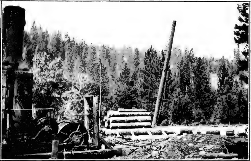
FIG. 1.—TYPICAL LANDING AND GIN-POLE USED FOR LOADING IN THE SUGAR PINE REGION.
