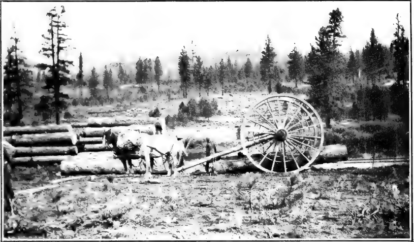
FIG. 1.—A PAIR OF STIFF-TONGUE BIG WHEELS AT THE LANDING, READY TO UNLOAD.
