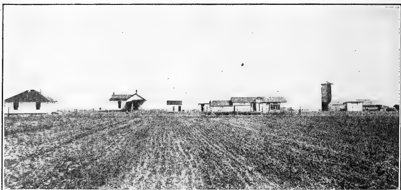
FIG. 2.—Buildings on the Cheyenne Experiment Farm, Archer, Wyo., in 1915. (Photograph lent by the Office of Dry-Land Agriculture Investigations.)
