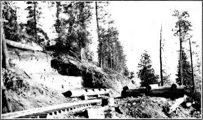
FIG. 1.—MAIN LINE LOGGING RAILROAD AND DUG LANDING ON TYPICAL LOGGING OPERATION IN THE SUGAR AND YELLOW PINE REGION.
