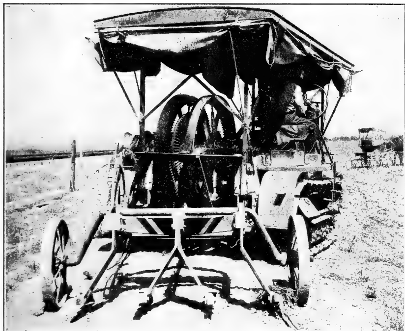
FIG. 16.—A 4-row beet harvester (side lifter) that is operated by a gasoline tractor.
