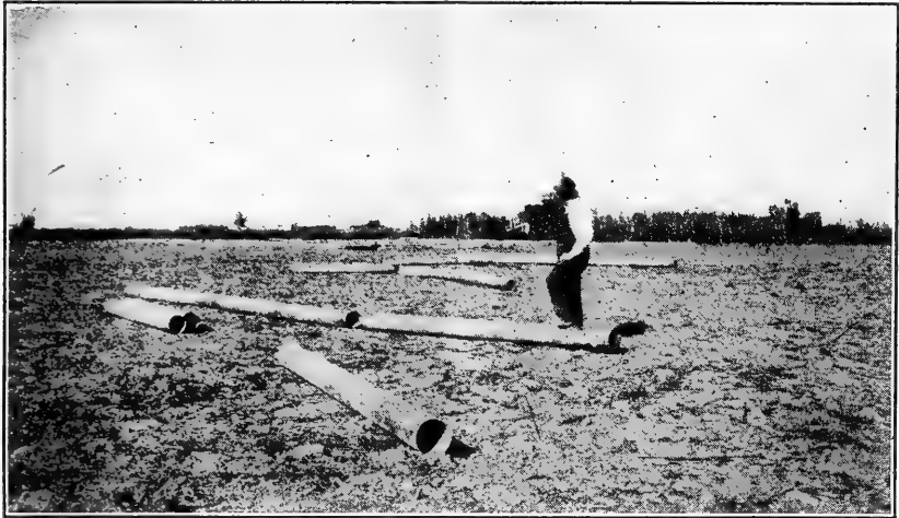
FIG. 12.—Pipes used for irrigating. They have been distributed across the field, but have not been connected in a continuous line.
