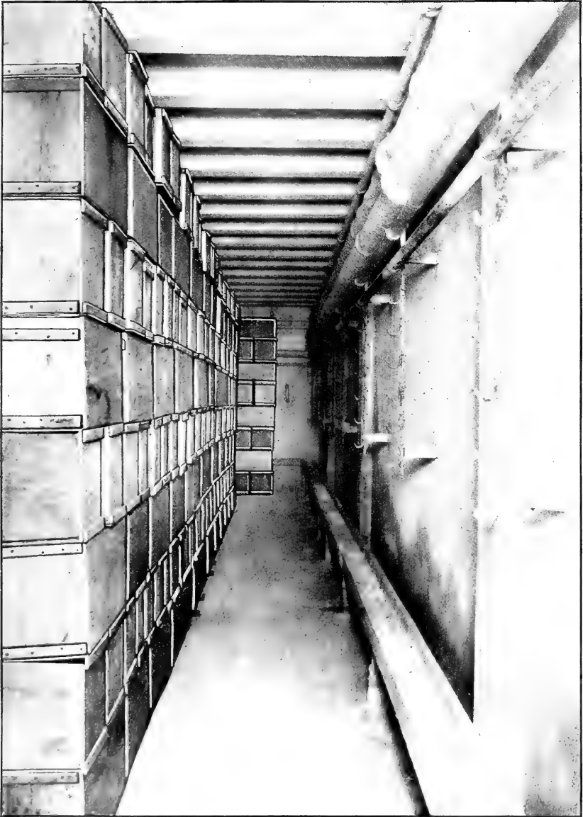
COLD-STORAGE ROOM, SHOWING BRINE COILS AND STACKS OF STORAGE-PACKED EGGS. CAPACITY, 4,000 CASES, OR 1,440,000 EGGS.
