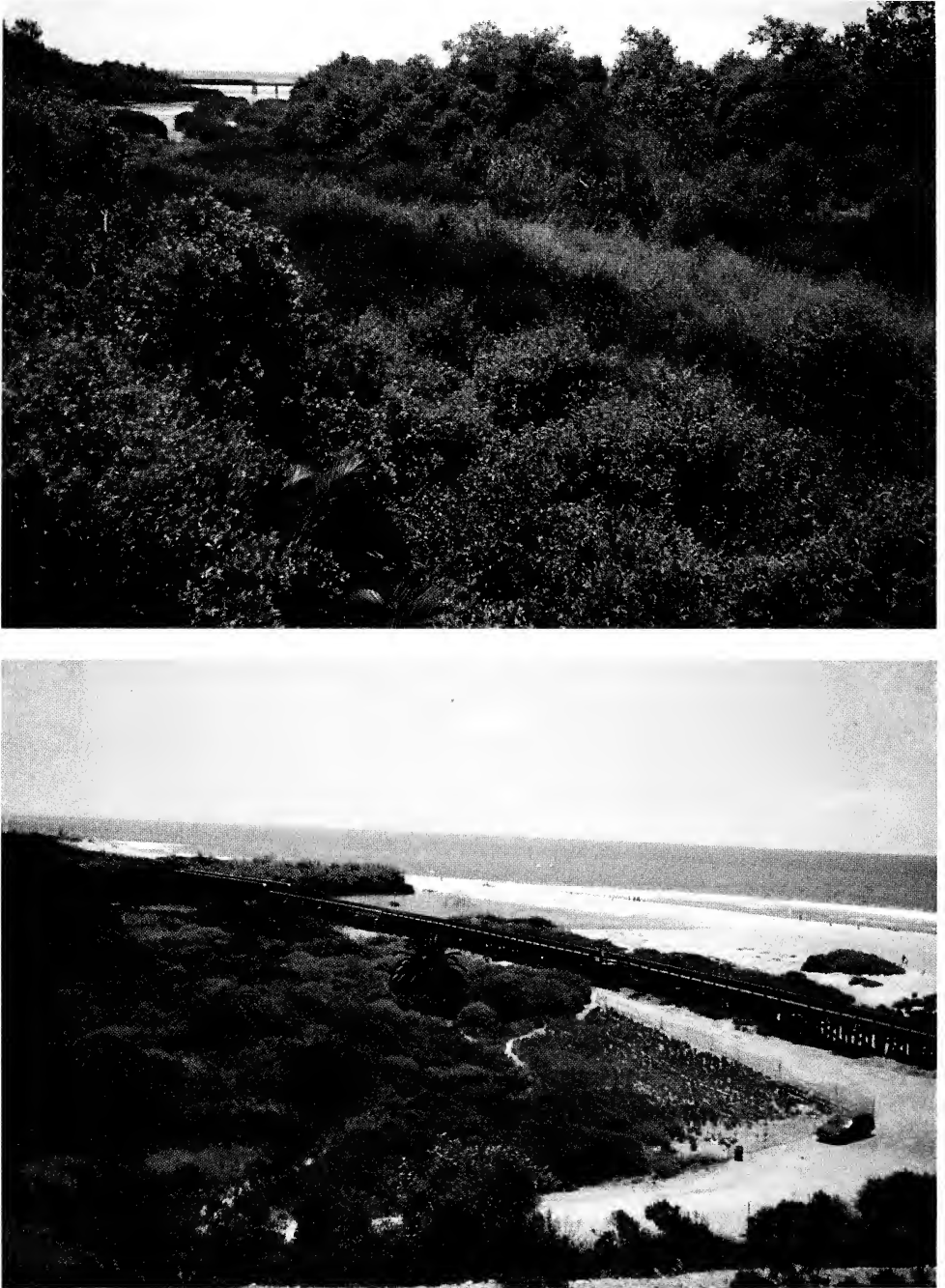
Fig. 4. San Mateo Lagoon. Upper: Downstream view of lagoon from Old Road Bridge; Lower: Lagoon mouth from north. Increased vegetation and closed to the ocean. 29 June 2000.
