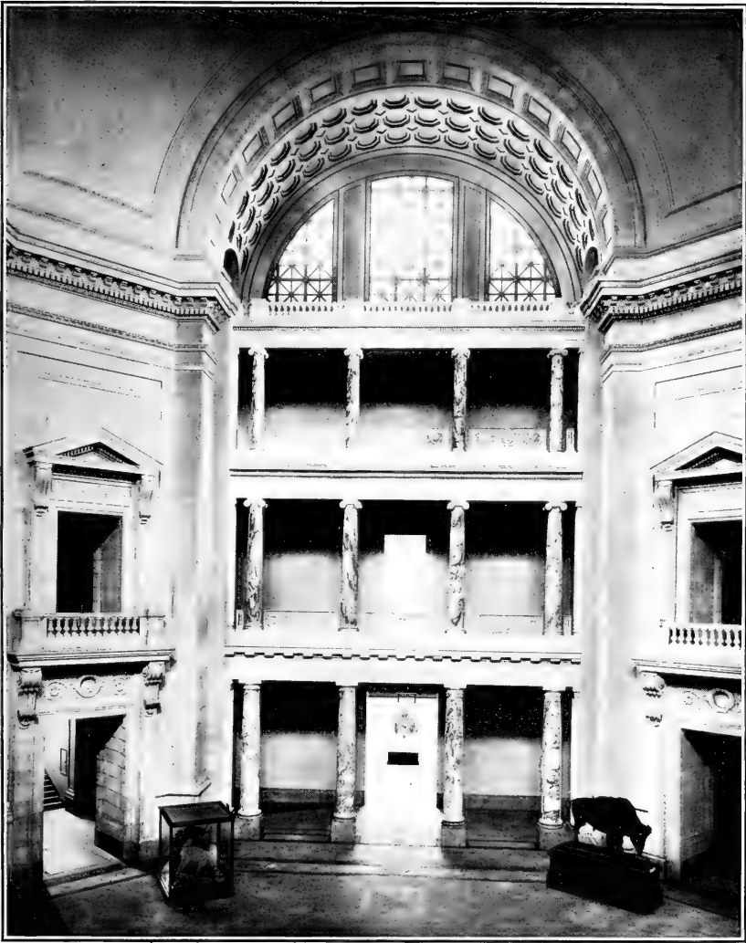
INTERIOR OF THE SOUTH PAVILION AND ROTUNDA TO THE HEIGHT OF THE TOP OF THE GREAT ARCHES, SHOWING THE SCREEN, WALLS, AND CLEARSTORY WINDOW ON THE EAST SIDE, AND PARTS OF THE ADJOINING STONE PIERS.
