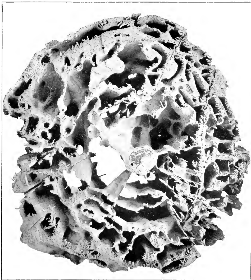
DAMAGE BY KALOTERMES HUBBARDI TO RAFTERS IN "ADOBE" BUILDING IN ARIZONA.
