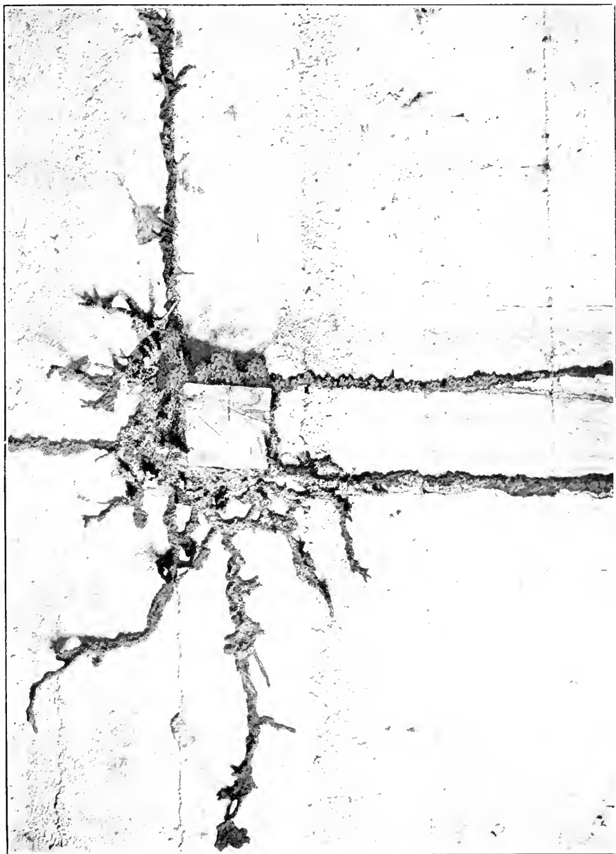
TUBES CONSTRUCTED BY RETICULITERMES HESPERUS ON WALL OF INFESTED BUILDING. LOS ANGELES, CALIFORNIA.
