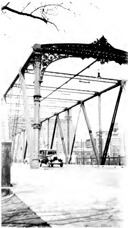
Figure 15.—NORTH STREET (now Guilford Avenue) bridge, Baltimore. In this transitional composite structure cast iron was used only in the relatively short sections of the upper chord. For the long unsupported compression members of the web system, standard wrought-iron angles and channels were built up into a large section. The decorative cast-iron end posts were non-structural. (Photo in the L. N. Edwards Collection, Museum of History and Technology.)
