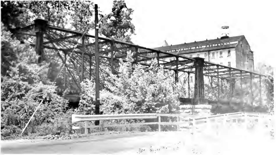
Figure 23.—THE ONLY SURVIVING BOLLMAN TRUSS BRIDGE, at Savage, Maryland. The bridge was built elsewhere in 1852 and was moved to this now-abandoned Baltimore and Ohio industrial siding in about 1898.
