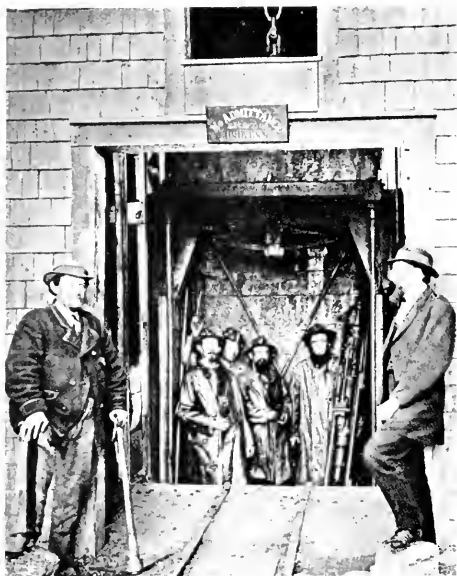
FIGURE 7.—HOOSAC TUNNEL. GROUP OF MINERS descending the west shaft with a Burleigh drill. (Photo courtesy of State Library, Commonwealth of Massachusetts.)
