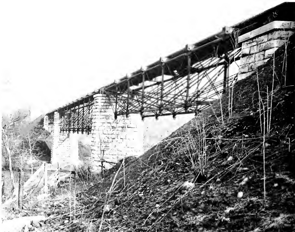
Figure 22.—BOLLMAN DECK TRUSSES in the North River Bridge built in 1873 at Mount Crawford, Virginia, on the Valley Railroad of Virginia (B. & O.). Each end span is 98 ft. 6 in.; the river span is 148 ft. 9 in. (Photo 756, Baltimore and Ohio Collection, Museum of History and Technology.)
