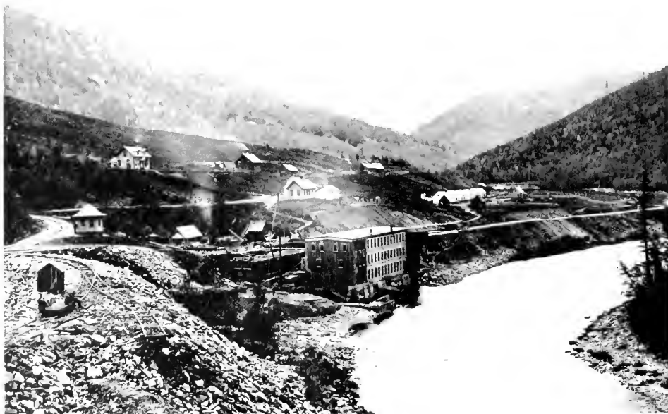
Figure 13.—HOOSAC TUNNEL. AIR-COMPRESSOR BUILDING on Hoosic River near North Adams. The compressors were driven partially by waterpower, derived from the river. ( Photo courtesy of State Library, Commonwealth of Massachusetts. )
