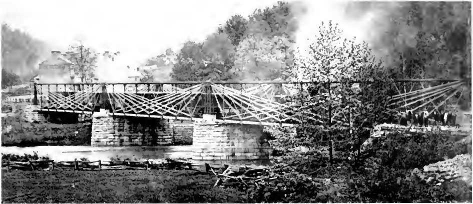
Figure 9.—BOLLMAN SKIOW BRIDGE at Elysville (now Daniels), Maryland, built in 1853-1854. (Photo courtesy of Maryland Historical Society.)
