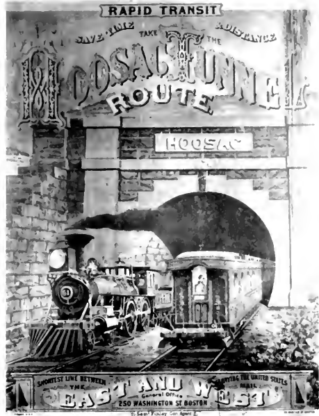
Figure 16.—WEST PORTAL UPON COMPLETION, 1876. (Photo courtesy of New-York Historical Society.)
