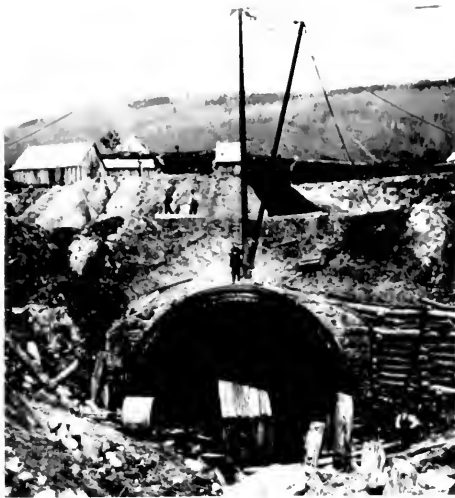
Figure 14.—WEST PORTAL OF HOOSAC TUNNEL before completion, 1868, showing six rings of lining brick.
