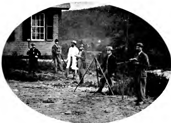
Figure 11.—HOOSAC TUNNEL survey crew at engineering office. The highest accuracy of the aboveground and underground survey work was required to insure proper vertical and horizontal alignment and meeting of the several separately driven sections. (Photo courtesy of State Library, Commonwealth of Massachusetts.)
