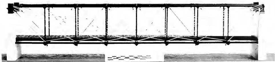
Figure 7.—RECENT MODEL of Bollman's Winchester span. Only two of the three lines of trussing are shown. The model is based on Bollman's published description and drawings of the structure. (USNM 318171; Smithsonian photo 46041.)
