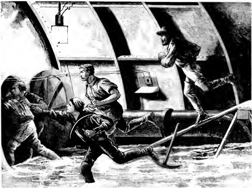
Figure 40.—ARTIST'S CONCEPTION OF MINERS escaping into the air lock during the blowout in Haskin's tunnel
