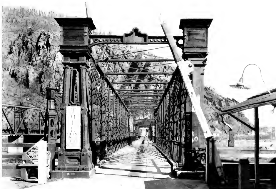
Figure 21.—The HARPERS FERRY BRIDGE toward the end of its career, carrying a common road over the Potomac. The westernmost line of trussing and span no. 1 had been removed long before. View through the Winchester span looking toward Maryland in 1933. (Photo courtesy of Harpers Ferry National Historical Park.)
