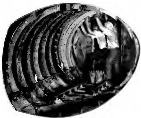
Figure 29.—PLACING A segment of cast-iron lining in Greathead's Tower Subway, 1869. To the rear is the shield's diaphragm or bulkhead. MHI model—1½" scale. (Smithsonian photo 49260 B.)
