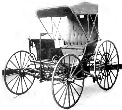
FIGURE 1. DURYEA AUTOMOBILE in the Museum of History and Technology, from an 1867 photograph. The gear-sprockets were already missing when this was taken, and the chain lies loosely on the pinion. Shown at the right, the Duryea vehicle following the recent restoration (Smithsonian photo 31483).
