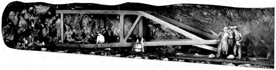
Figure 3.—HOOSAC TUNNEL. WORKING OF LATER STAGES with Burrell pneumatic drills mounted on carriages. The bottom heading is being drilled in preparation for blasting out with nitroglycerine. M.I.T. model \frac{1}{2} " scale. (Smithsonian photo 49260-M.)
