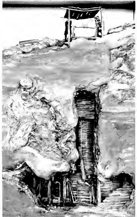
Figure 17.—SOFT-GROUND TUNNELING. The support of walls and roof of mine shaft by simple timbering; 16th century. MHH model— \frac{3}{4} " scale. (Smithsonian photo 49260-J.)
