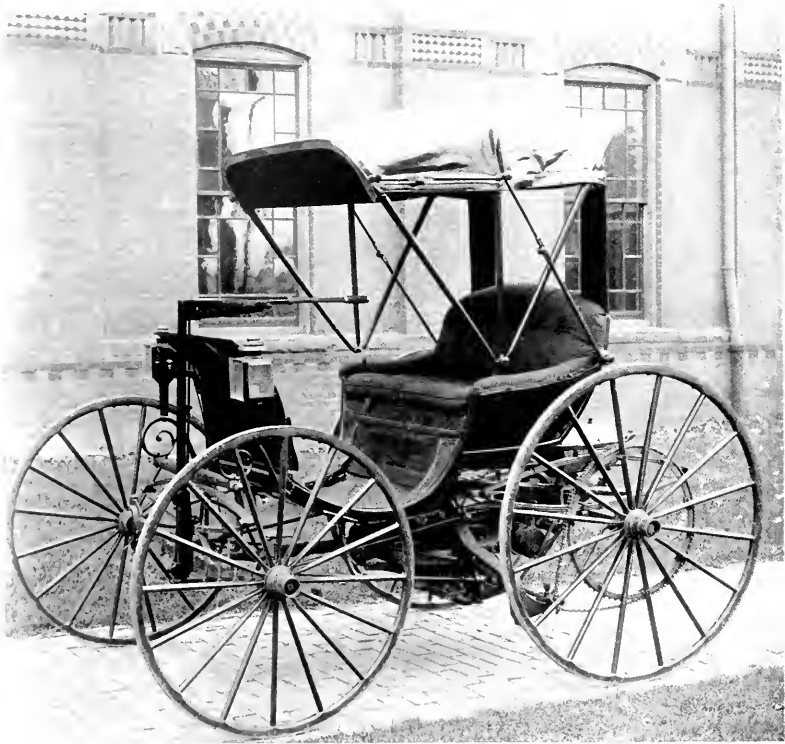
FIGURE 1. DURYEA AUTOMOBILE in the Museum of History and Technology, from an 1867 photograph. The gear-sprockets were already missing when this was taken, and the chain lies loosely on the pinion. Shown at the right, the Duryea vehicle following the recent restoration (Smithsonian photo 31483).
