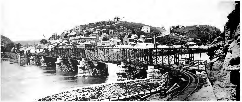
Figure 13.—THE FOUR BOLLMAN SPANS at Harpers Ferry that survived the Civil War. The spans were completed in 1862-1863. (Photo courtesy of Baltimore and Ohio Railroad.)
