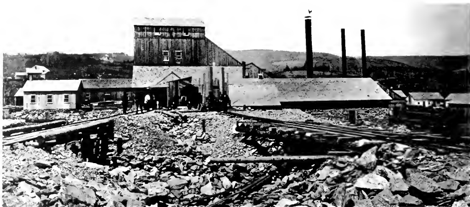
Figure 12.—WORKS AT THE CENTRAL SHAFT, HOOSAC TUNNEL, for hoisting, pumping and air compressing machinery, and general repair, 1871. ( Photo courtesy of State Library, Commonwealth of Massachusetts. )
