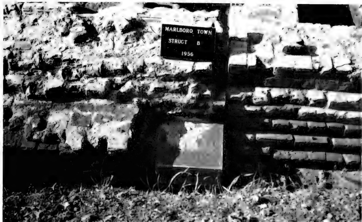
Figure 34.—SOUTHWEST CORNER OF STRUCTURE B. Plain, unglazed, red sandstone block at junction of junction of main foundation wall and sign, molded red-sandstone trim can be seen in background. Bricks in front of trim appear to have been added later as step foundation. Base of main-foundation footing appears at right.
