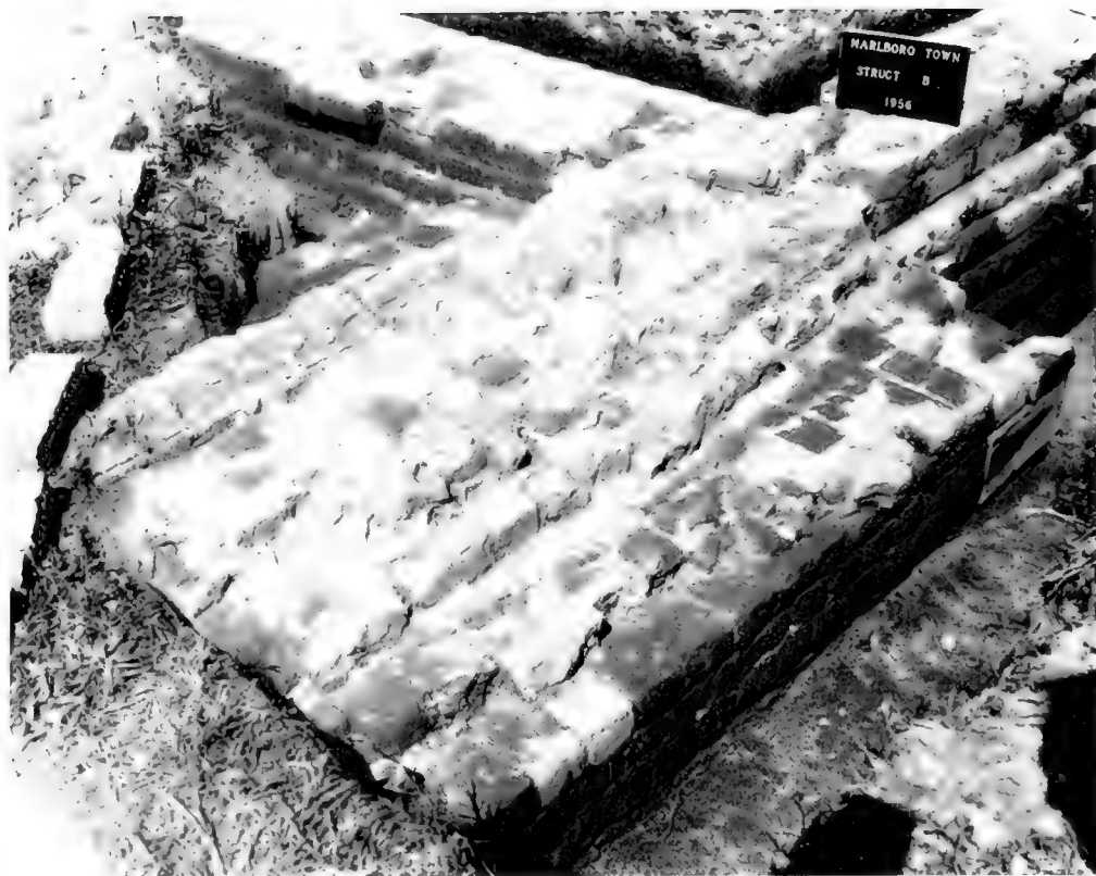
Figure 35.—SOUTHWEST CORNER OF STRUCTURE B, showing molded-sandstone trim with added brickwork in front. Bricks also covered red-sandstone block, lower right. (Diagonally placed bricks at left are not part of structure.)
