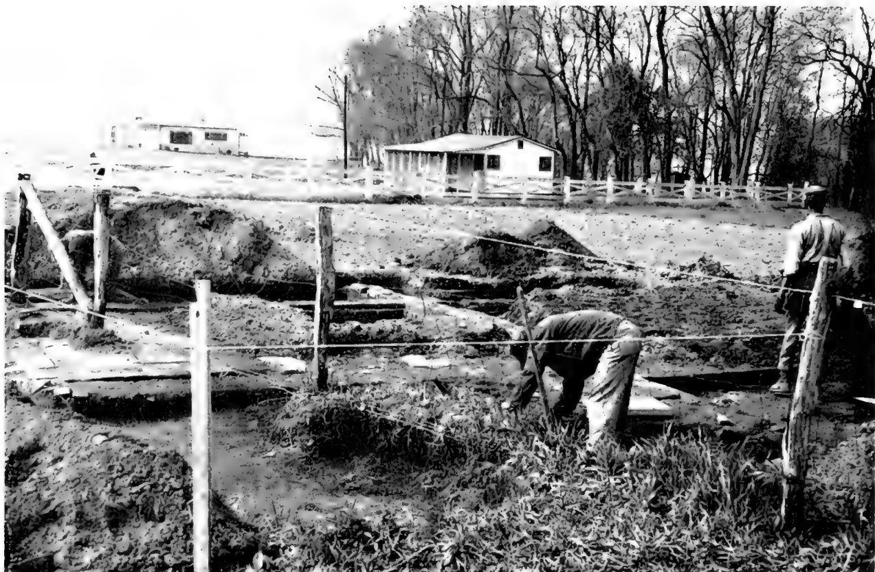
Figure 47. FOUNDATION of Structure E (kitchen).
