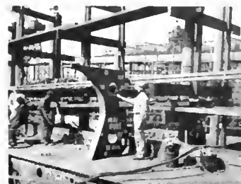
A Web Frame Is Set and Fitted
