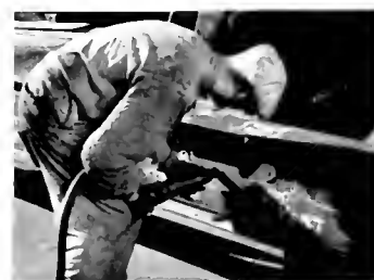
Driving High Tensile Rivets
