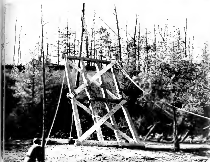
2. High trestle for bridge is too heavy for lifting, so a derrick is rigged.
