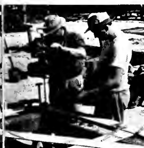
Spaul is clamped together and drilled if it is drilled for bolting
