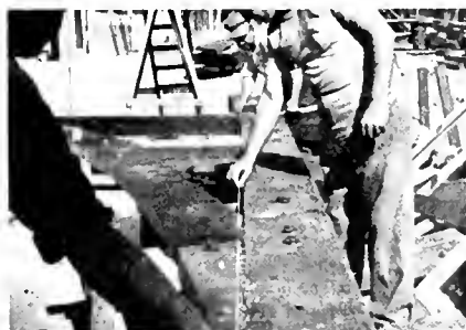
After bolting, all reference lines are accurately marked
