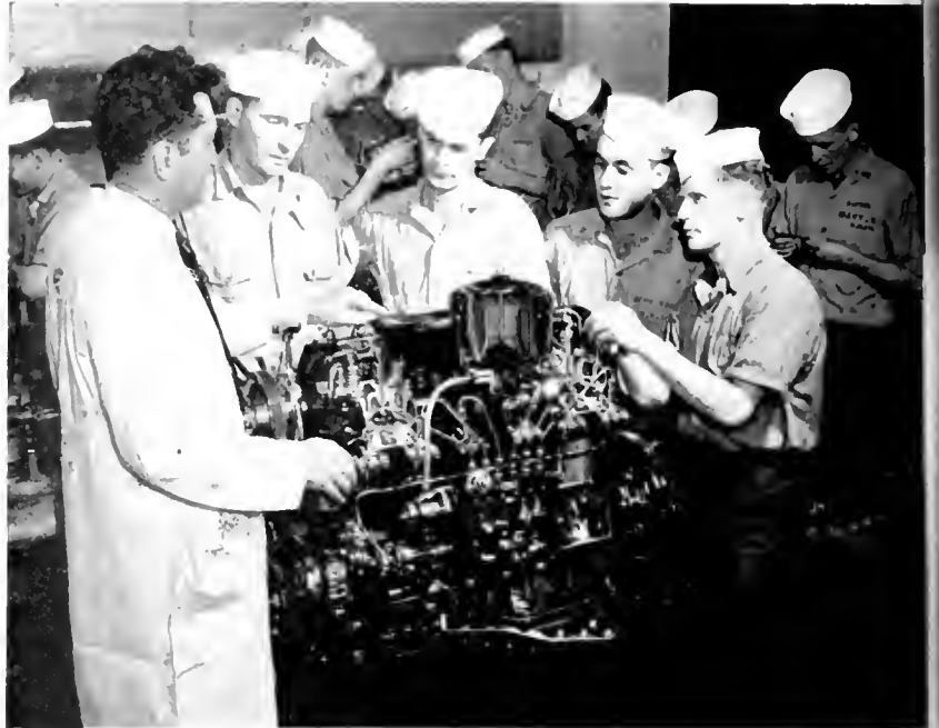
Cut-away models allow students to see and understand the inner mechanism of equipment.
