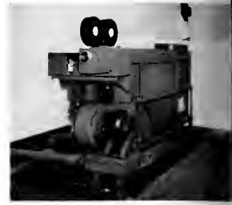
General view of camera-developer viewer equipment, AN/GRD-1. (PERL)
