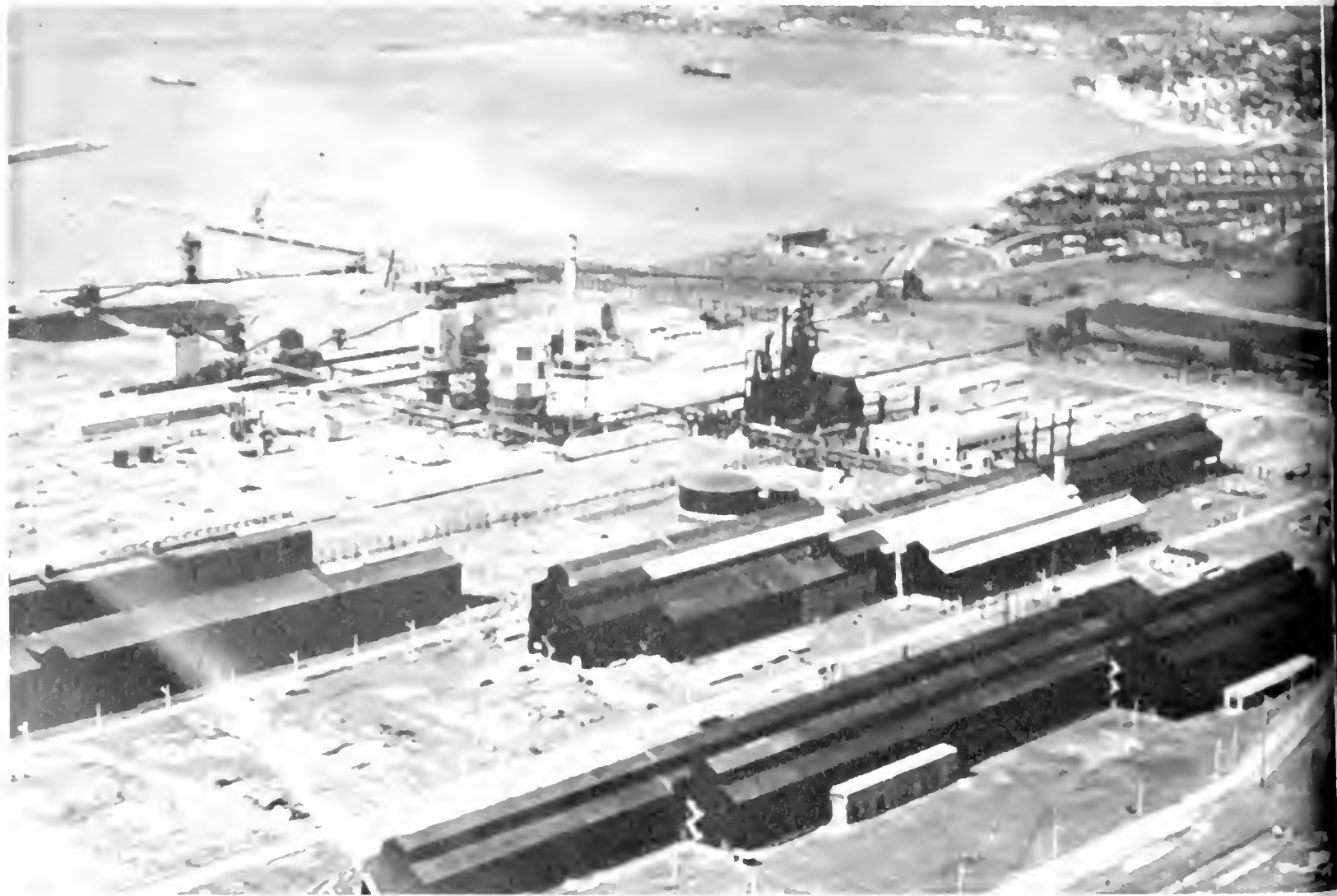
This aerial view, looking toward the Black Sea, shows the completed steel plant located one mile southwest of city of Ereğli, shown in upper right corner.
