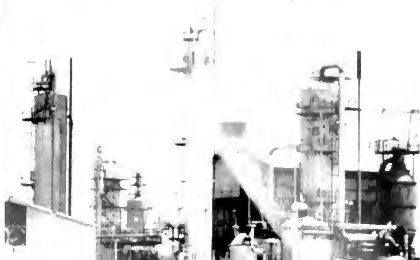
Among Armour Chemical Company's far-flung facilities pictured in sales film "The Vertagreen Story" is scene of its nitrogen plant at Cherokee, Ala.
