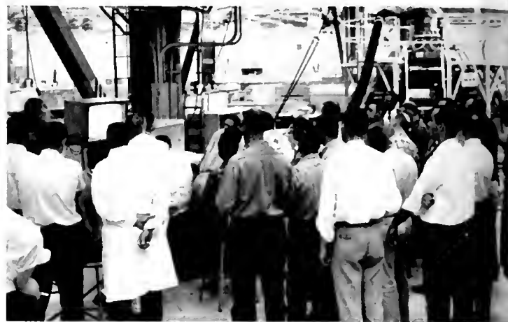
Monitors in working areas enable employees to view closed-circuit television.
