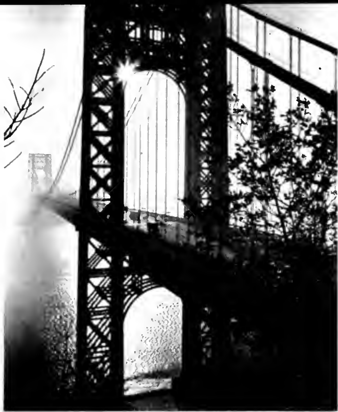
The George Washington Bridge beckons visitor to Manhattan
