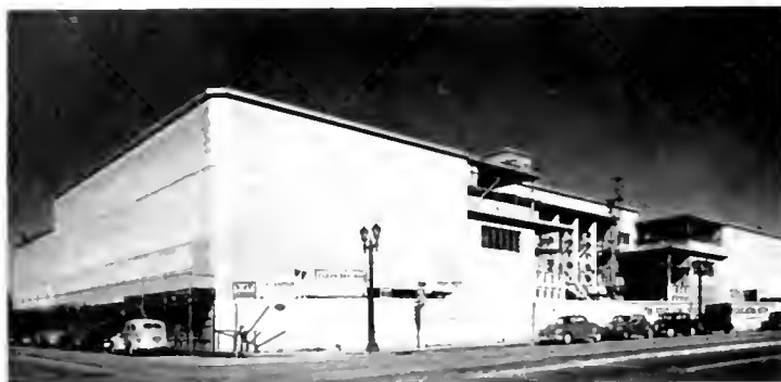
MODERN FUNCTIONAL DESIGN FEATURES the KHL, Don Lee Broadcasting Studio building nearing completion in Hollywood this month.
