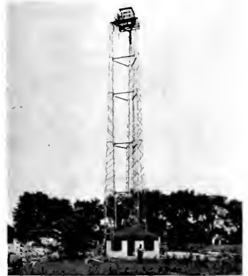
This relay tower at Michigan City is one of two stations along the 90-mile "bridge".
