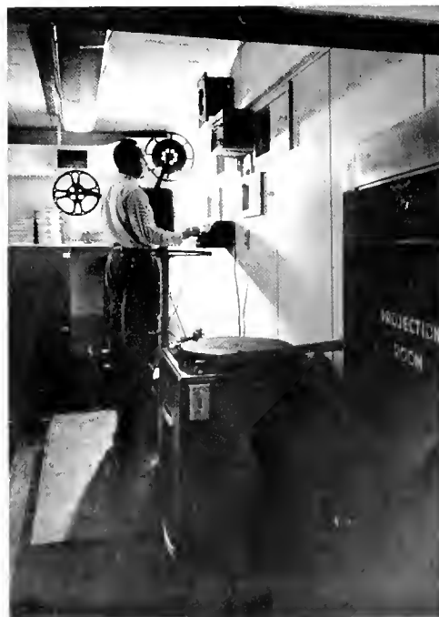
Projection room in operation. Operator has hand on volume control. Note monitoring speaker overhead. On small shelf between ports is inter-com unit used for talking to conference room telephone. Projector operator is D. G. Lovell, film librarian.
