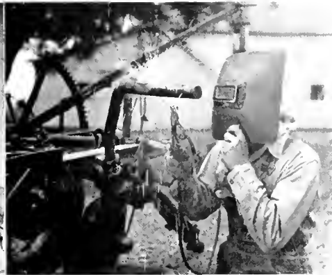
Rebuilding a worn plow with welding in scene from Wilding film for Lincoln Electric Company.
