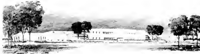
NEW VICTOR ANIMATOGRAPH CORPORATION PLANT in Davenport, Iowa, as visualized by architect. Construction is planned to begin in 1948 on site already selected.
