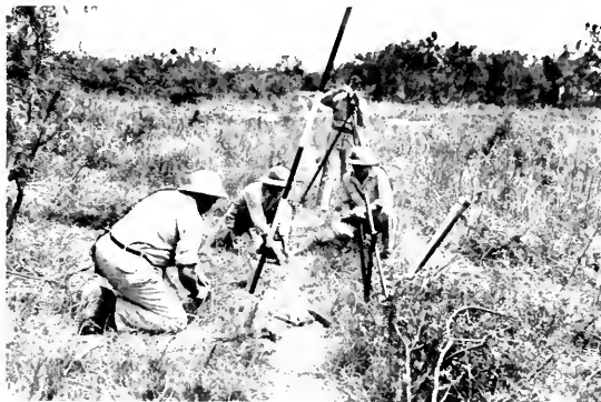
The surveying crews lay out a line which will be followed by the seismic crews "earthquakers" who set off small charges to get a picture of the underground rock structure—as shown in "10,000 Feet Deep."
