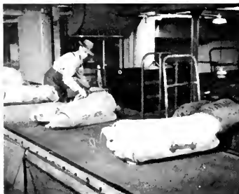
ENDLESS CONVEYOR BELT on which incoming mail is loaded. Each position down the belt takes a bag, separates by destination.
