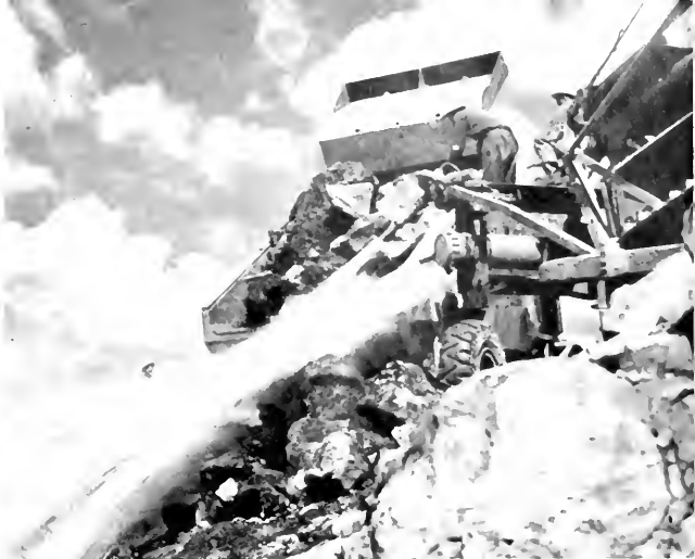
TRUCKLOADS OF ROCK are dumped on the growing wall of the huge Kenney Dam where high-pressure streams of water wash away loose material and help bind rock surfaces of the world's largest clay-core dam.
