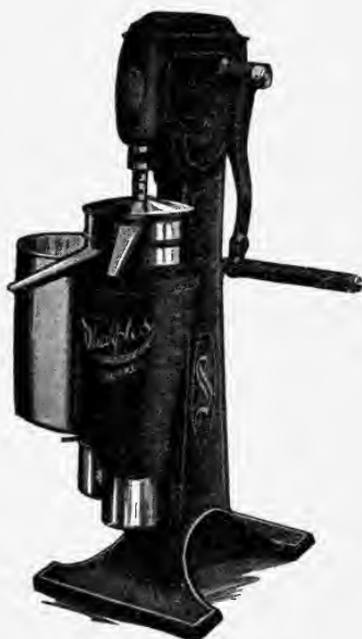
Fig. 10. Sharples hand separator Courtesy Sharples Separator Co.
