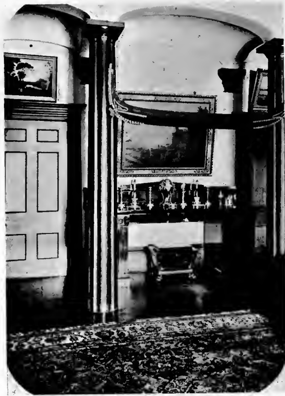
Fluted Ironbark Columns. Camden House, N.S.W.
