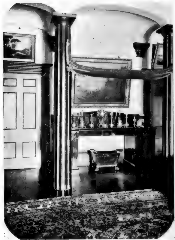
Fluted Ironbark Columns. Camden House, N.S.W.
