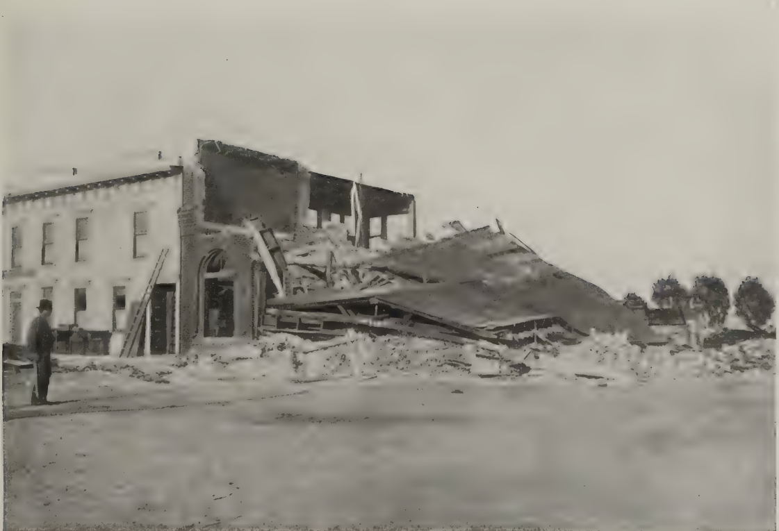
B. Wreck of 2-story brick building, San Mateo. Per J. C. B.
