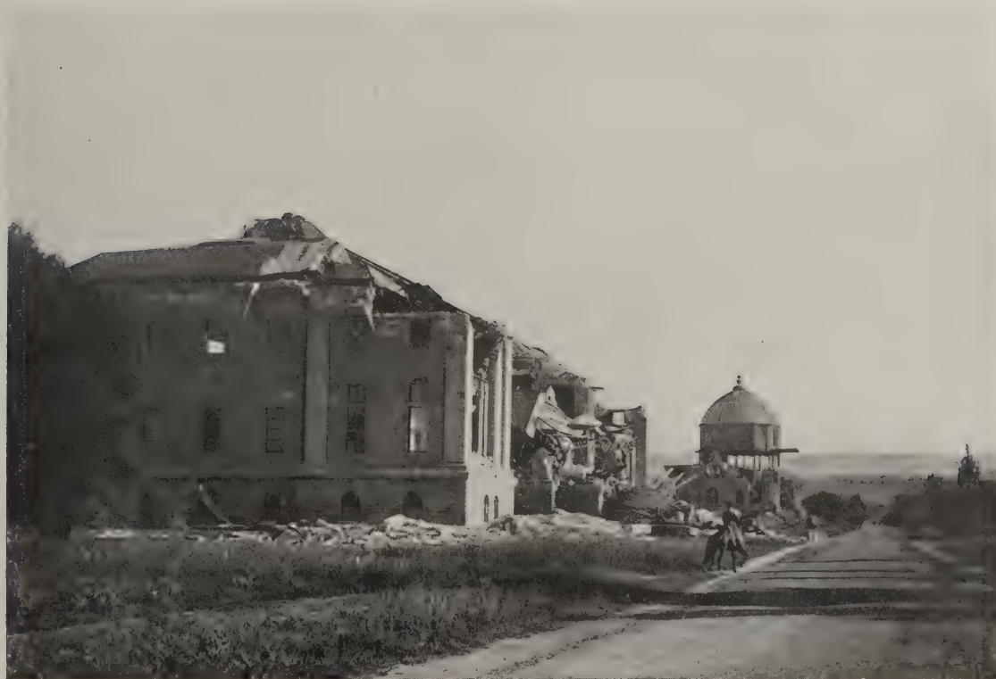
B. Wreck of Gymnasium Building, Stanford University. Per J. C. B.
