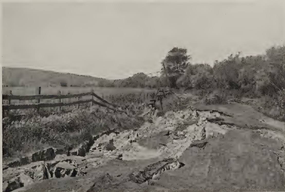
B. Destruction of road due to lurching of ground toward Salinas River. Near Spreckels. A. C. L.
