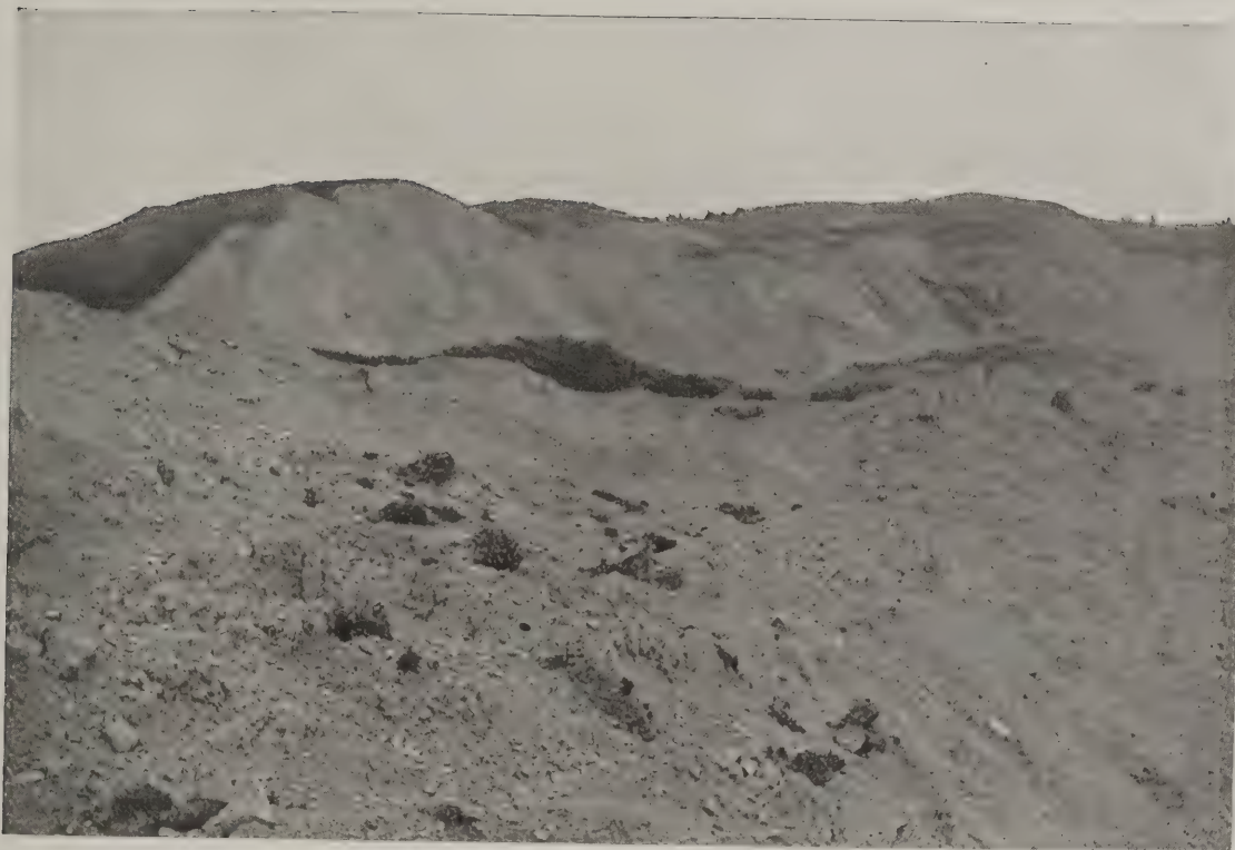
A. Earth-slump at Cape Fortunas, Humboldt County. A. S. E.
