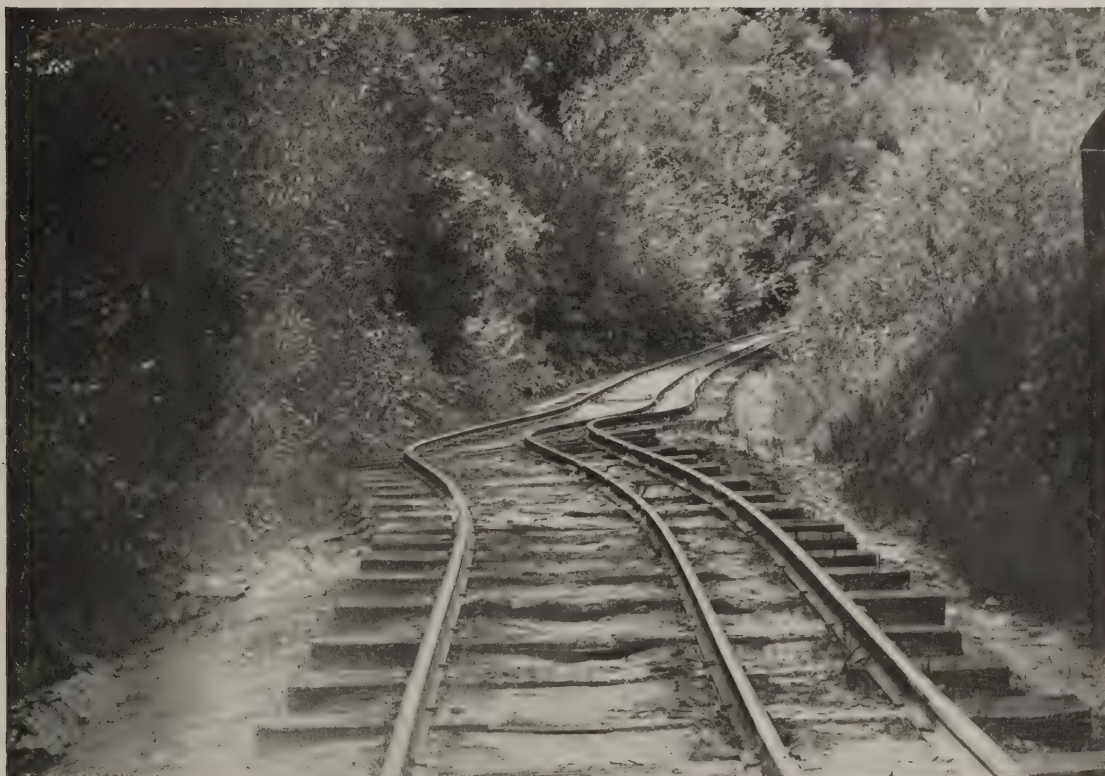
A. Shortening of railroad track between Los Gatos and Santa Cruz. G. A. W.
