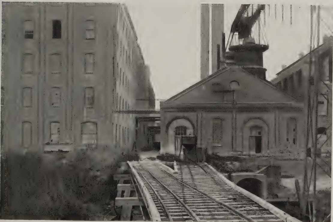
B. Spreckels sugar mill. Looking northwest. A. C. L.
