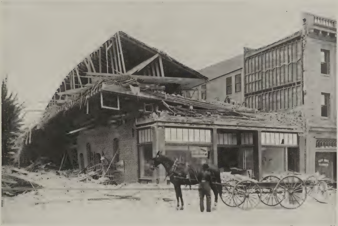
A. Wreck of 2-story brick building, San Mateo. Per J. C. B.
