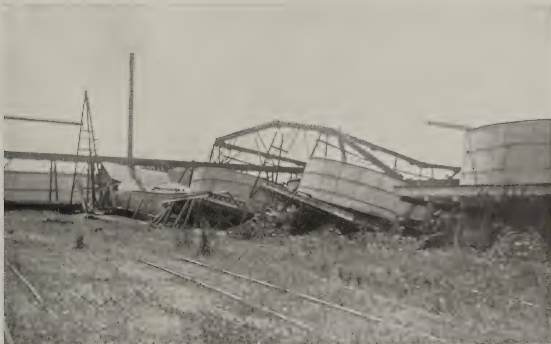
A. Alvarado. Wreck of molasses tanks, Alameda Sugar Company. E. W. B.
