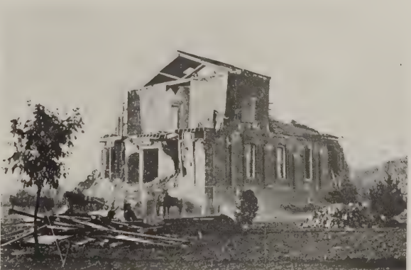
F. Court-house, San Leandro. Wrecked by earthquake of 1868.
