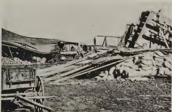
C. Flour mill and warehouse, Haywards. Wrecked by earthquake of 1868.
