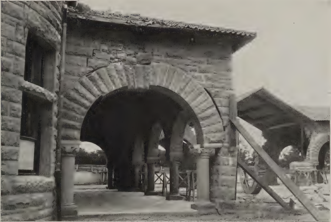
A. Wrecked arches, Geology Building, Stanford University. Per J. C. B.
