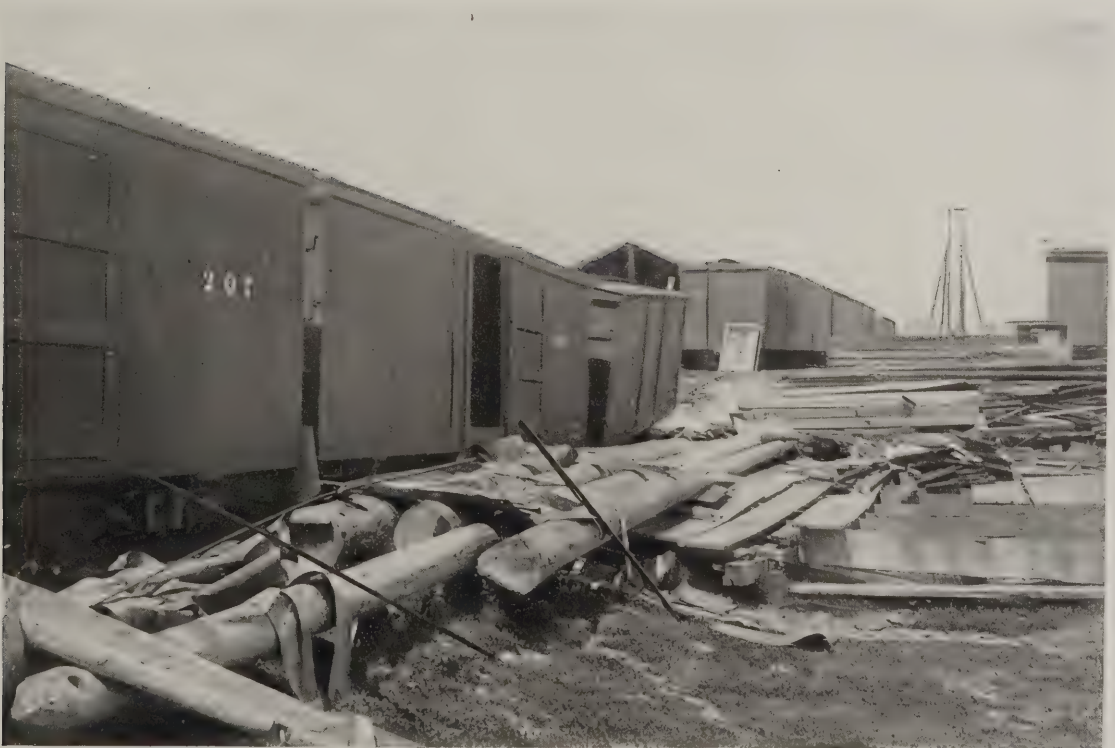
B. Moss Landing. Deformation of surface due to lurching of ground toward Salinas River. A. C. L.
