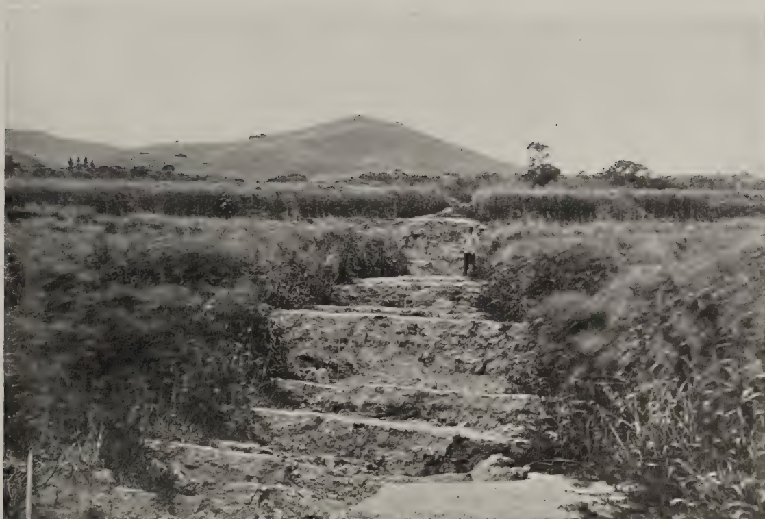
A. Lurching of ground toward Salinas River, with consequent collapse. Near Spreckels. Per J. O. B.
