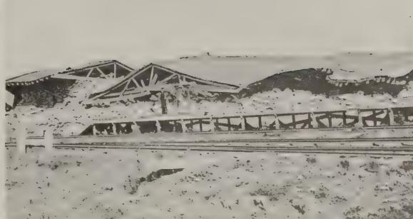
B. Edmonson's warehouse, Haywards. Wrecked by earthquake of 1868.
