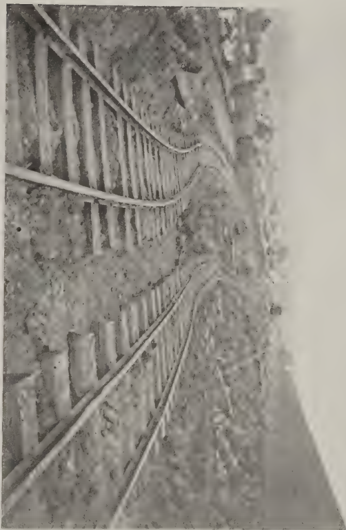
A. Earth-slump north of Tomales, carrying railway roadbed with it. Track was straight before earthquake. R. S. H.
