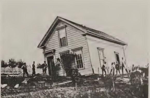
D. Pierce's house, Haywards. Earthquake of 1868.
