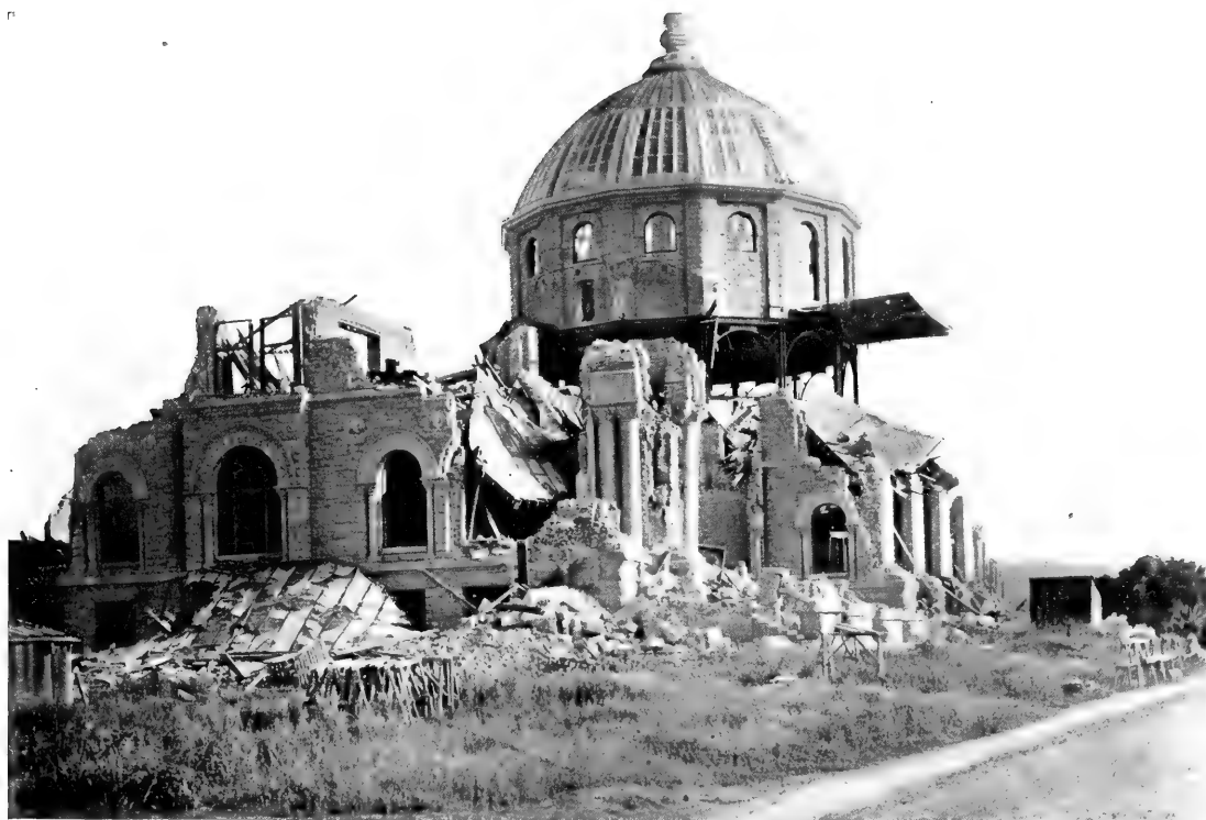
A. Wreck of Library Building, Stanford University. Per J. C. B.
