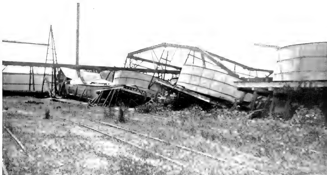
A. Alvarado. Wreck of molasses tanks, Alameda Sugar Company. E. W. B.
