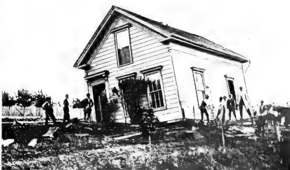
D. Pierce's house, Haywards. Earthquake of 1868.
