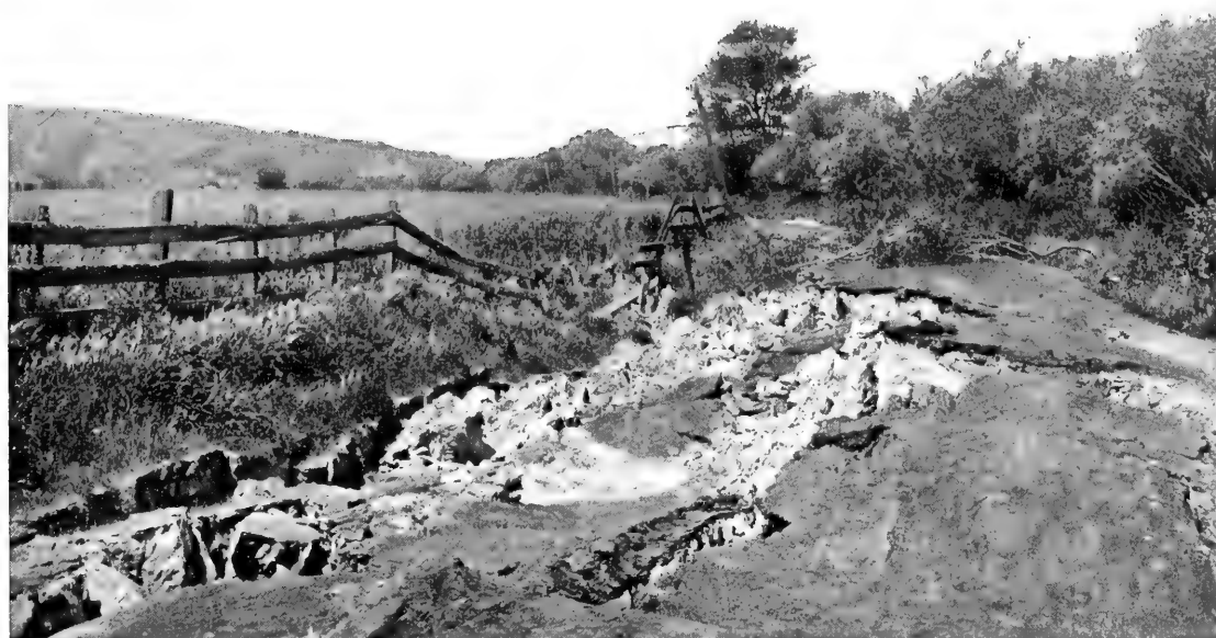
B. Destruction of road due to lurching of ground toward Salinas River. Near Spreckels. A. C. L.
