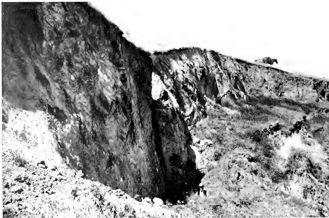
B. Scarp of landslide in southeast quarter of section 15, township 16 south, range 12 east, near Cantua. G. D. L.
