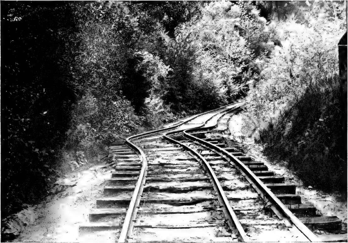
A. Shortening of railroad track between Los Gatos and Santa Cruz. G. A. W.
