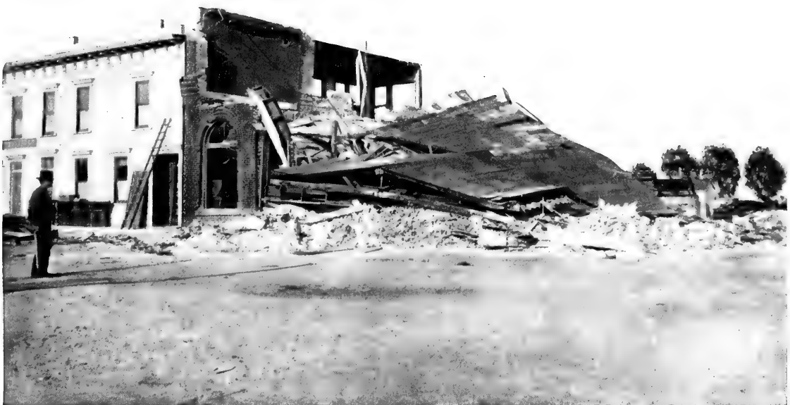
B. Wreck of 2-story brick building, San Mateo. Per J. C. B.
