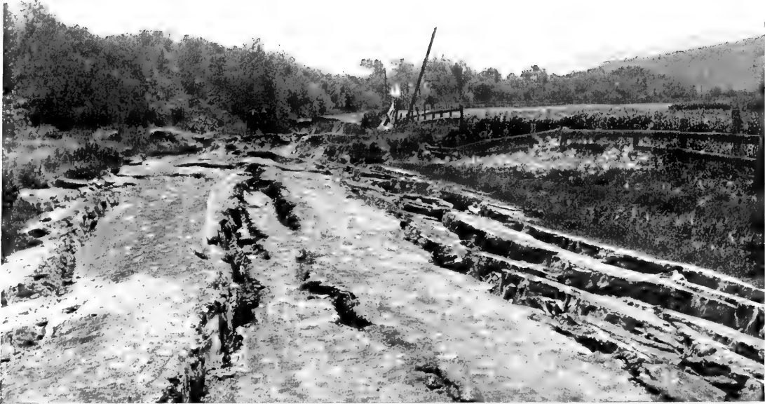
A. Lurching of ground toward Salinas River and consequent collapse. Near Spreckels. A. C. L.
