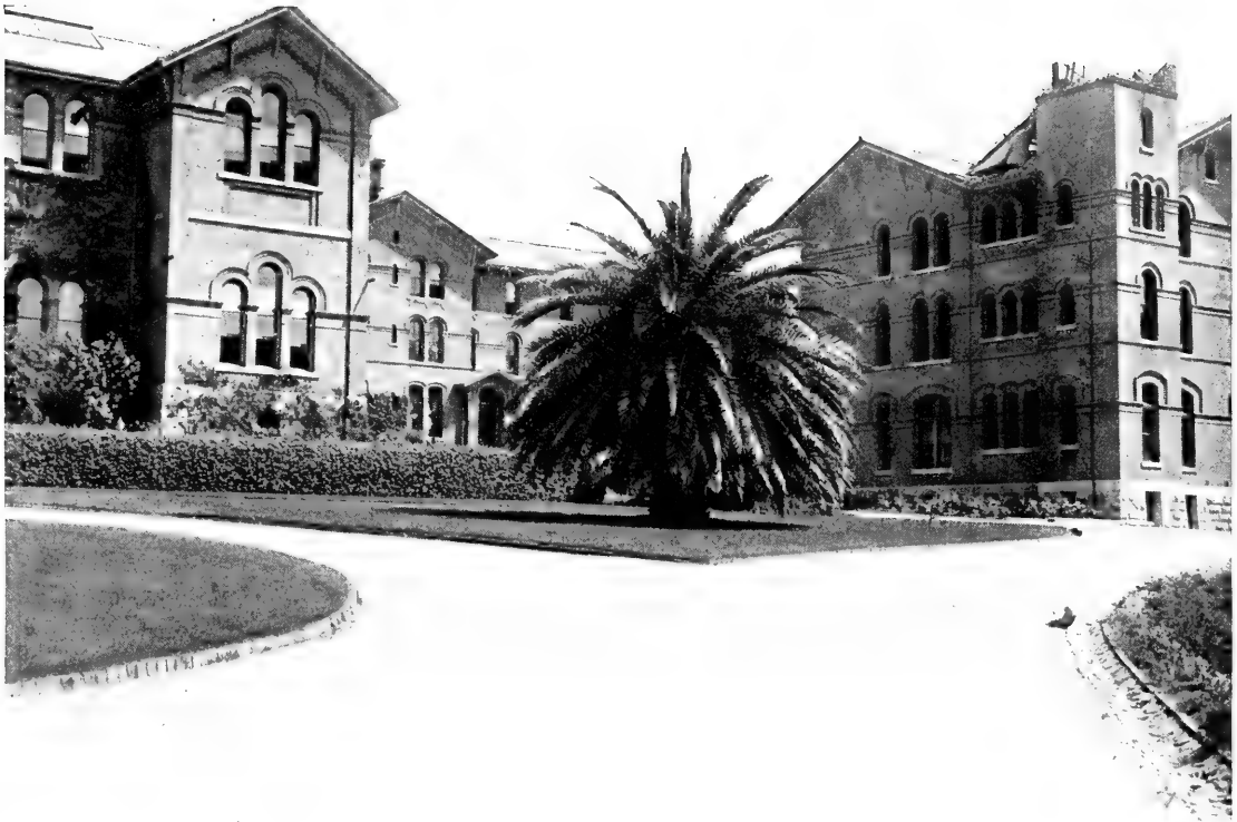
A. Berkeley. Institute for Deaf, Dumb, and Blind. South wing. A. C. L.
