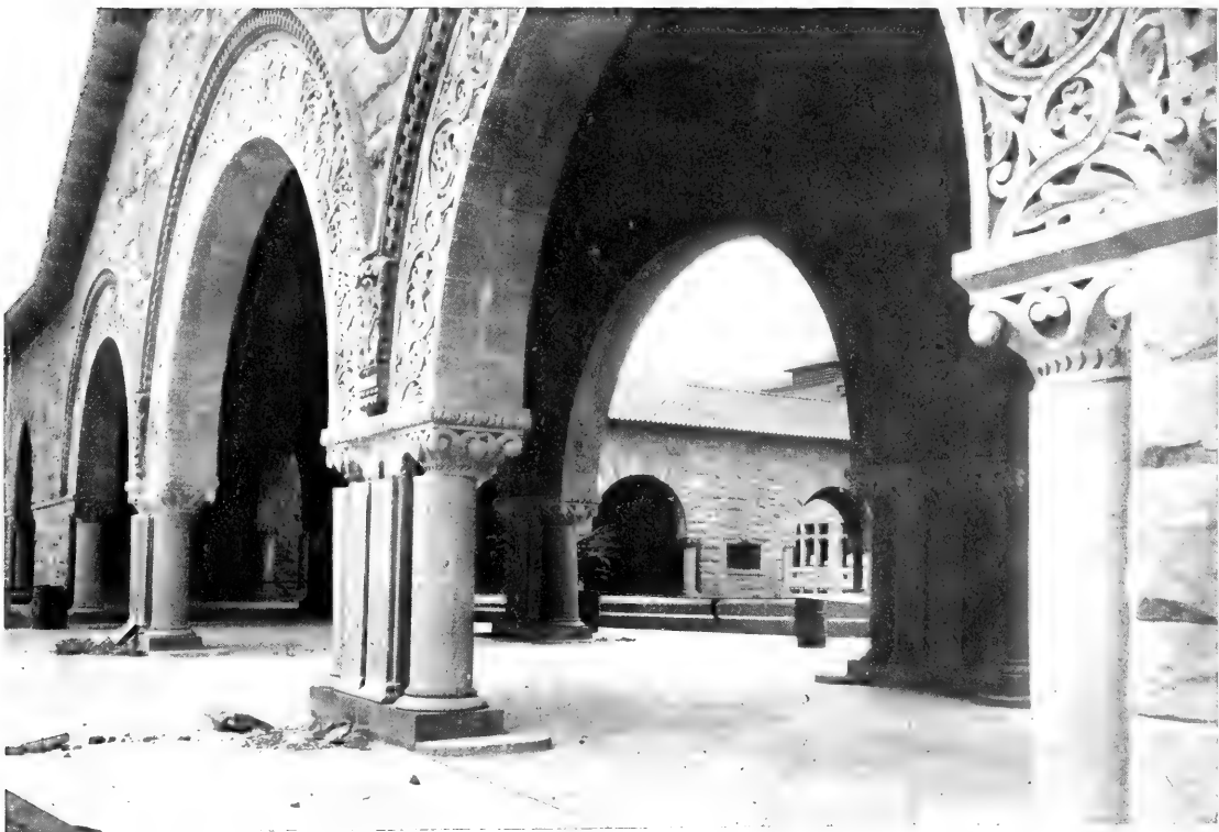
B. Arches that moved on their supporting columns, Stanford University. Per J. C. B.
