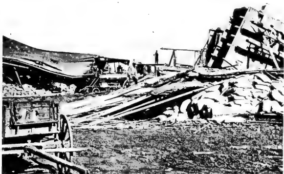
C. Flour mill and warehouse, Haywards. Wrecked by earthquake of 1868.
