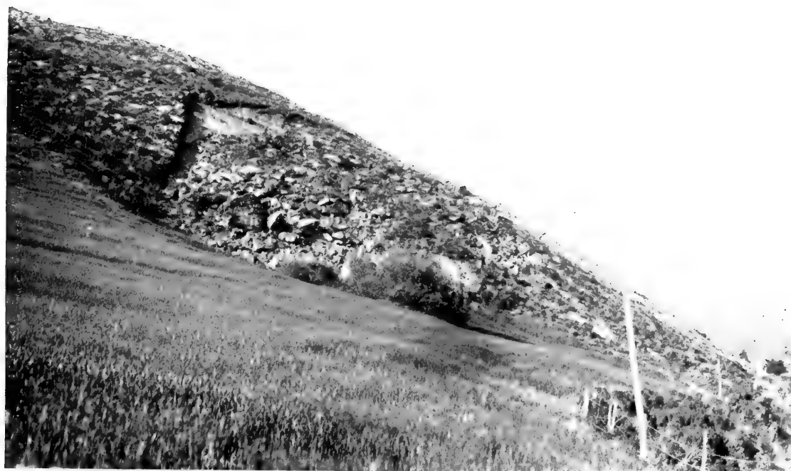
B. Earth-avalanche in sandstone near Half Moon Bay. Slip on bedding planes. E. D.
