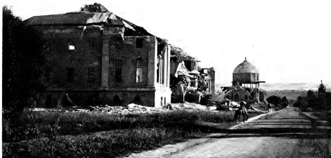
B. Wreck of Gymnasium Building, Stanford University. Per J. C. B.
