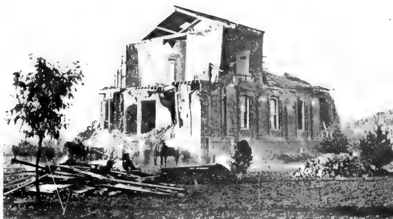
F. Court-house, San Leandro. Wrecked by earthquake of 1868.
