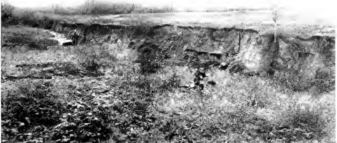
B. Secondary crack, with drop of 7 feet, in alluvial flood-plain of Pajaro River. G. A. W.
