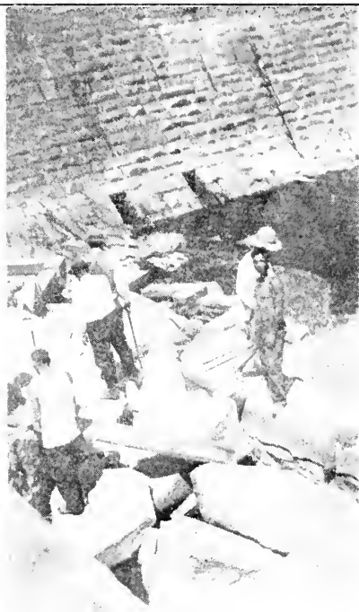
FIG. 100. Convicts working on fish ladder at Folsom dam. Dead eels in pool beyond. Photograph by G. I. Fleckenstein, July 2, 1928.
