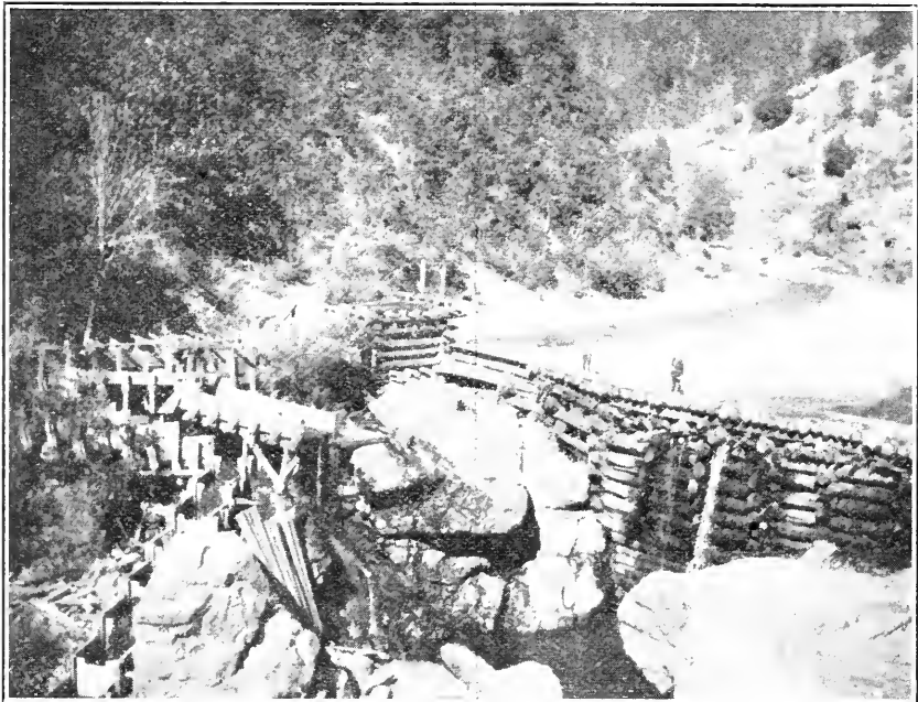
FIG. 31. McGillavray Dam on Canyon Creek, Trinity County, showing the new fish ladder recently completed. October, 1927. Photograph by G. O. Laws.
