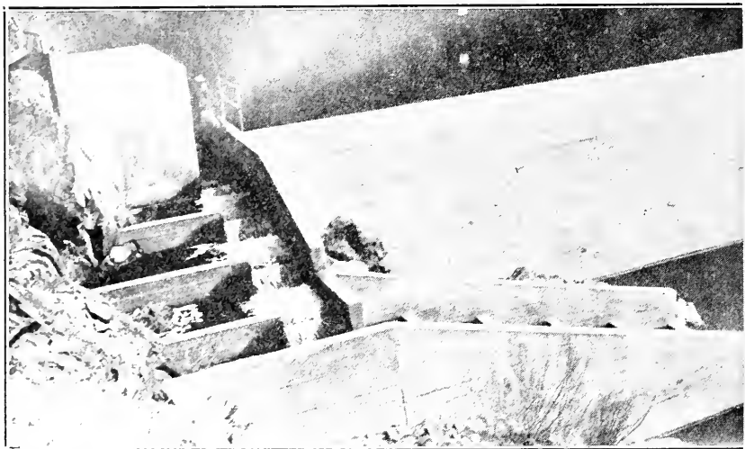
Fig. 55. Fishway of concrete construction. Natural rock bank forms bottom and portion of one side. A float at upper port regulates amount of water through fishway.
