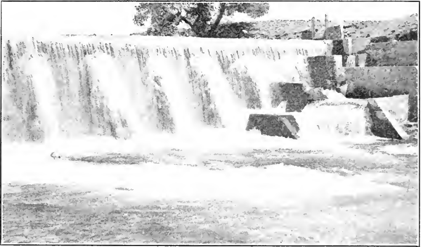
FIG. 17.—Fish ladder over Clough Dam on Los Molinos River, Shasta County, California. Similar fish ladders have been placed over practically all the important dams in the state, thus giving fish access to the headwaters of the streams.
