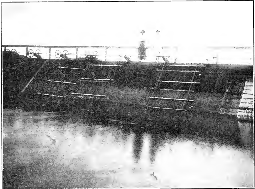
FIG. 18.—A partial view of the largest fish screen in the state. This screen, installed by the Sacramento Valley West Side Canal Company, in Glenn County, is seventy feet long and fifteen feet deep.
