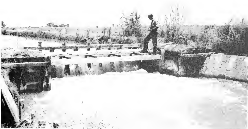
FIG. 82. A check on a canal in the Palo Verde Irrigation District. Fish congregate at such points. May 1942.
