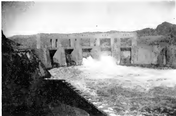
FIG. 53. Upstream view of Parker Dam. Foundation for power house on left. Photograph by D. A. Clanton, Jan. 25, 1939.
