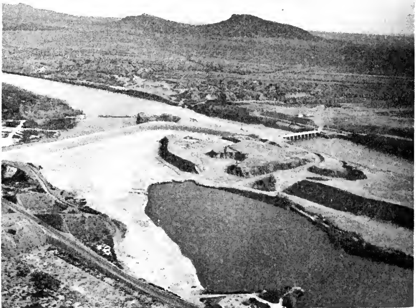
FIG. 52. Headgate Rock Diversion Dam, upstream view. Photograph through courtesy of U. S. Indian Service.
