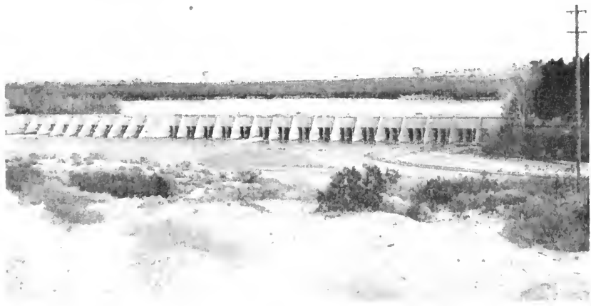
FIG. 49. Rockwood Gate, diversion point for the Alamo Canal. Upstream view. Jan. 1942.
