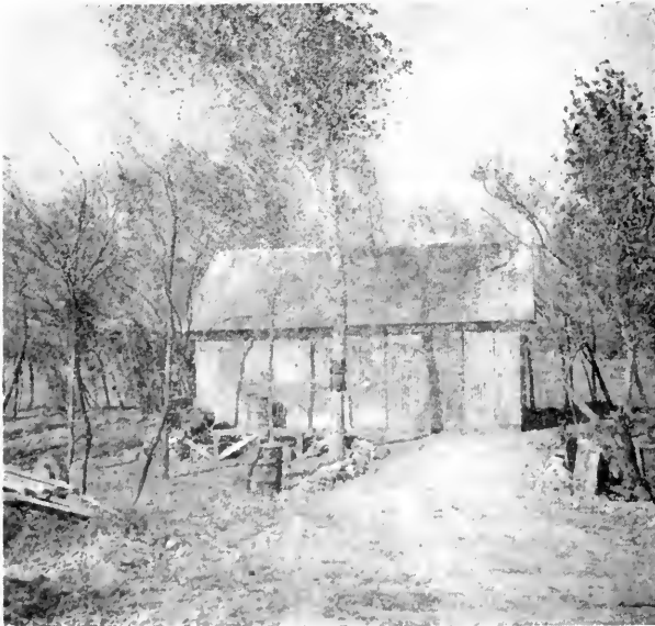
FIGURE 48. Portable storehouse located above Fort Mohave, Arizona, used for storage of equipment when not in operation.
