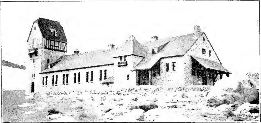
Fig. 32. Mt. Whitney Hatchery as it appears completed.
