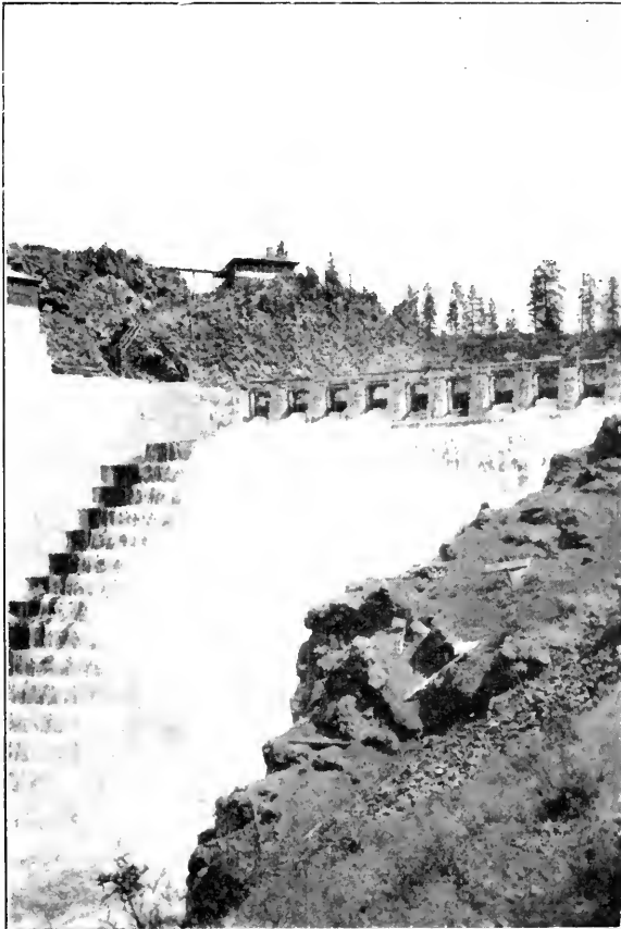
FIG. 40. Copco Dam on the Klamath River. This dam is so high that a fish ladder was not feasible. Consequently, the California-Oregon Power Company was compelled to build a fish hatchery in lieu of a fishway. Photograph by C. Westerfeld.
