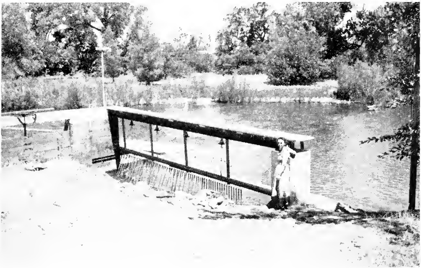
FIGURE 9. Mill Creek electric fish screen
