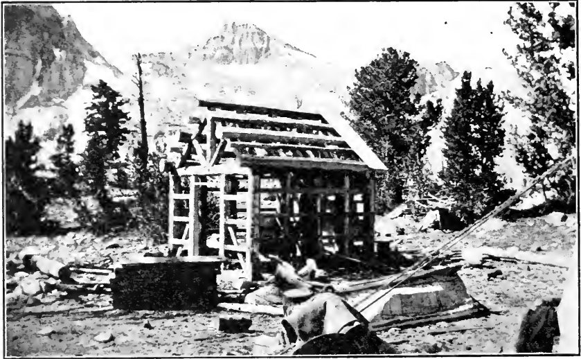
Fig. 50. New egg collecting station at Rae Lakes, showing the type of structure that must be erected to withstand the heavy snows at elevations above 10,000 feet. Photograph by F. H. Shebley.
