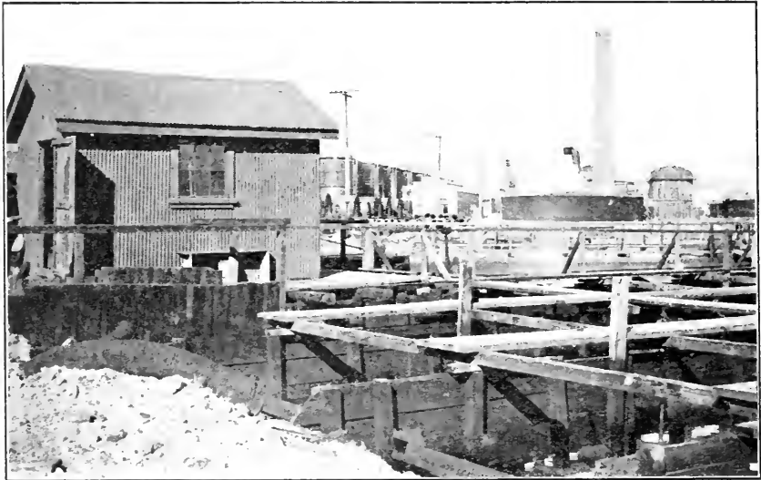
Fig. 76. Detail view of baffles of the Standard Oil Company plant at Richmond. The oil collects behind the baffles and is skimmed and pumped back into the separator. Photograph by A. M. Fairfield.
