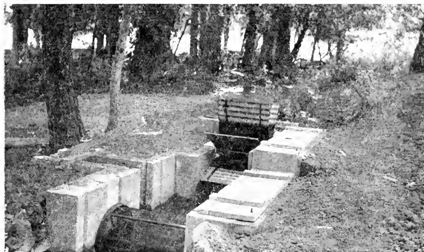
Looking upstream on a rotary fish screen. Power wheel in front of screen Opening in concrete wall at left is for flushing out moving sand and gravel
