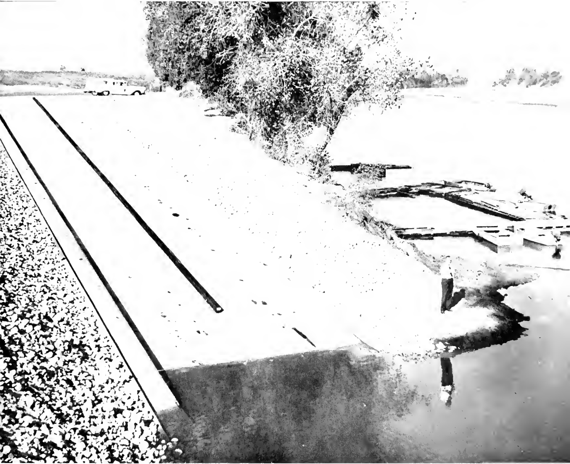
Typical of access sites provided by Wildlife Conservation Board funds is this one on the Feather River near Boyd's Pump. Under construction in the biennium, the ramp is 22 feet wide and has a two foot walkway down the left side. Boat docks were built by local sportsmen.
