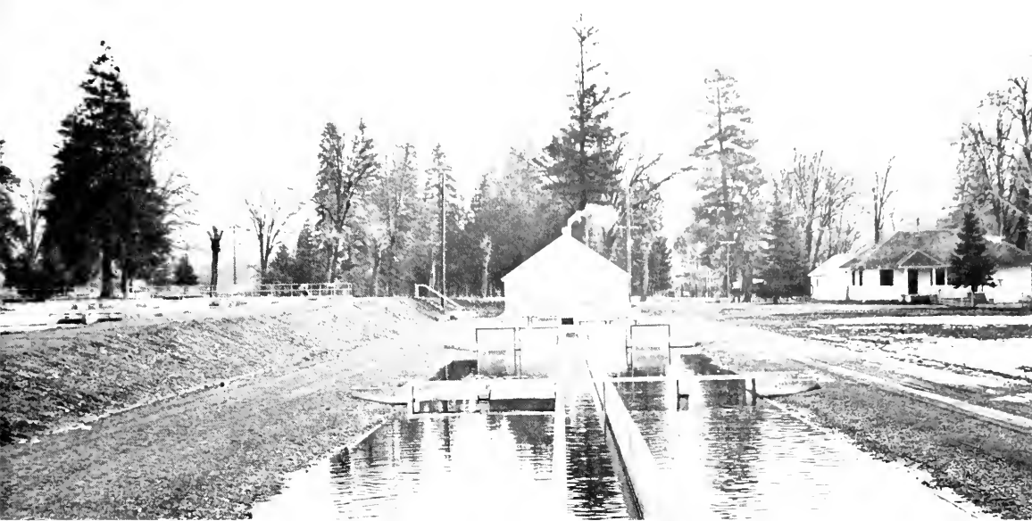
New brood stock ponds and spawning house at Mt. Shasta Hatchery. Fish are pushed into the spawning house without removing them from the water, resulting in less injury to the fish and better quality eggs taken.
