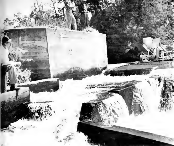
Fish ladders help salmon and steelhead to pass dams blocking passage to upstream spawning beds. —Fish and Game Photo
