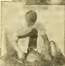
4. Tamp Soil Around Edge of Setter.
