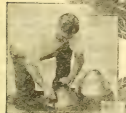
5. Remove Setter from HOTKAP. One Man Can Place 3,000 HOTKAPS per Day.
