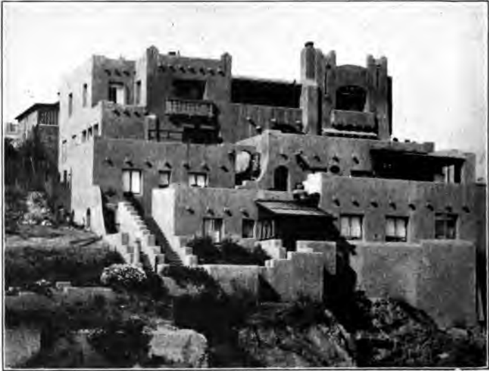
REBUILDING SAN FRANCISCO.
