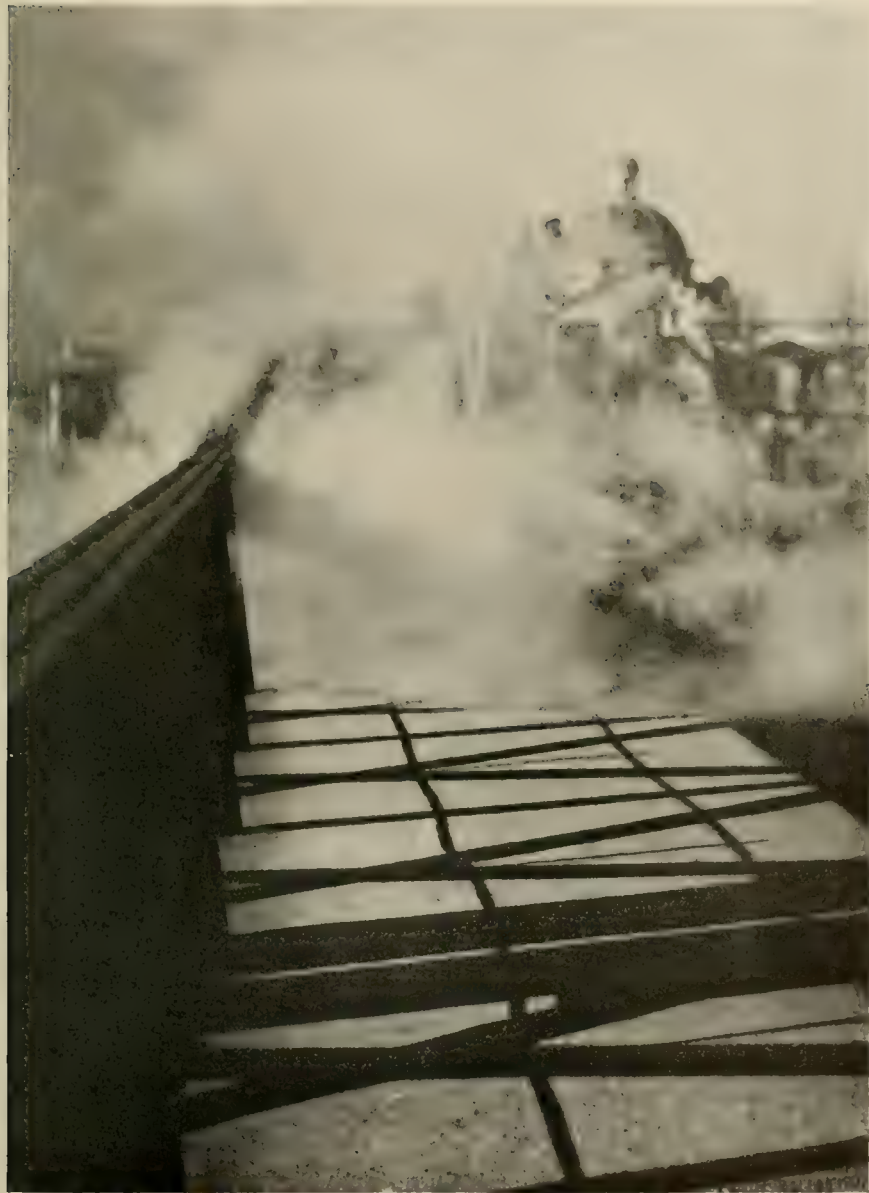
The Railway Bridge Guido Pellegrini
