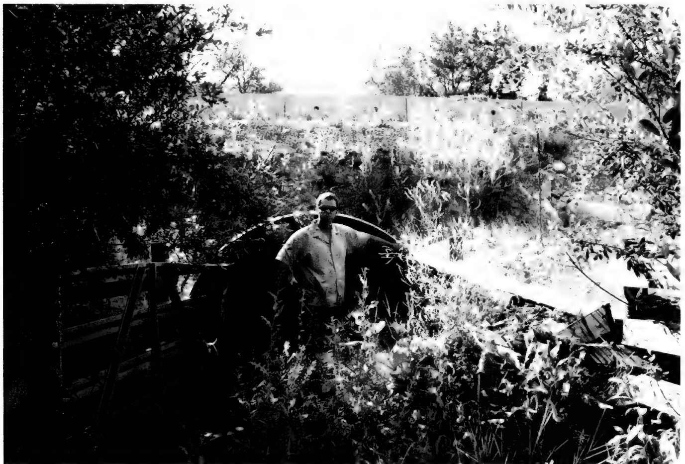
FIGURE 1. Drainage culvert at Site 1, used repeatedly by Mule Deer to travel under the Trans-Canada Highway near Kamloops, British Columbia (dimensions of culvert: 2.1 m wide, 1.5 m tall, 30 m long).
